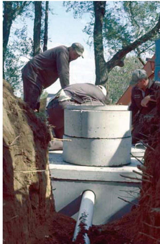
Workers install a new septic system.
