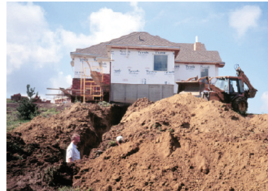
Soils are often disturbed during construction.
