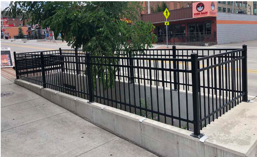
Tree trench on a steep slope in Ames, Iowa.
