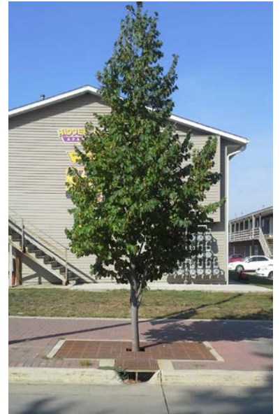
Examples of green inlets installed in Cedar Falls.
