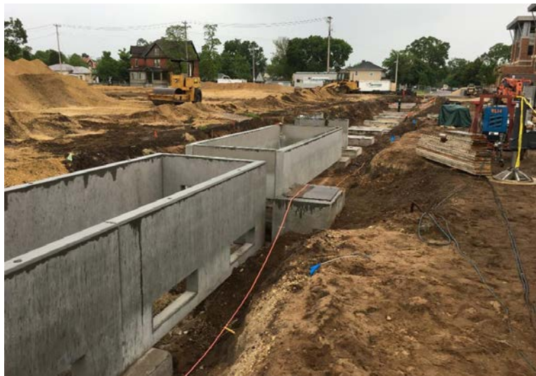
Precast planter boxes being installed in La Crosse, Wisconsin.
