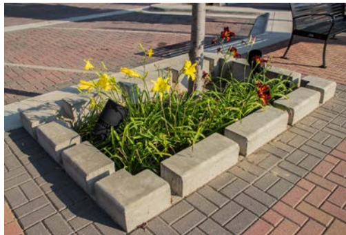
Small curb openings allow water to enter from sidewalk areas in Coralville, Iowa.
