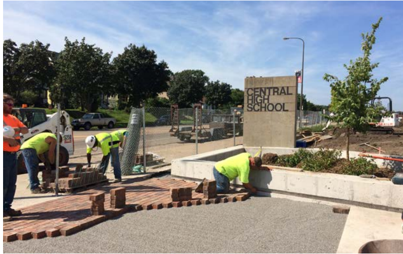
Permeable pavers being installed next to a planter box.
