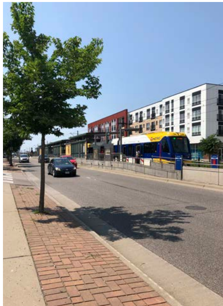
Tree trench installed under permeable pavers..
