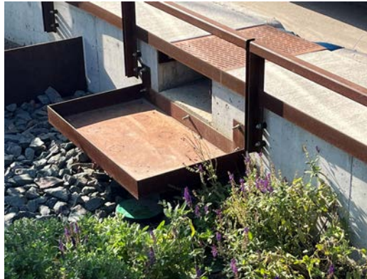
A metal edger is used as a pretreatment area at a curb cut at this location in Des Moines.
