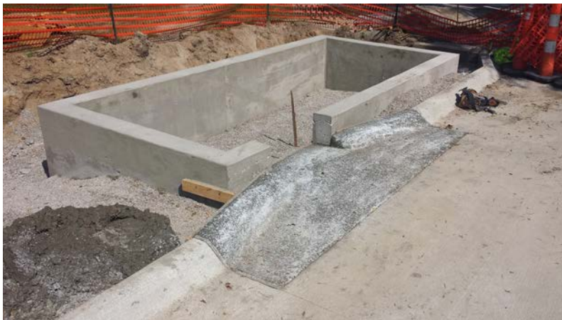
Cast in place planter box during construction in Coralville.
