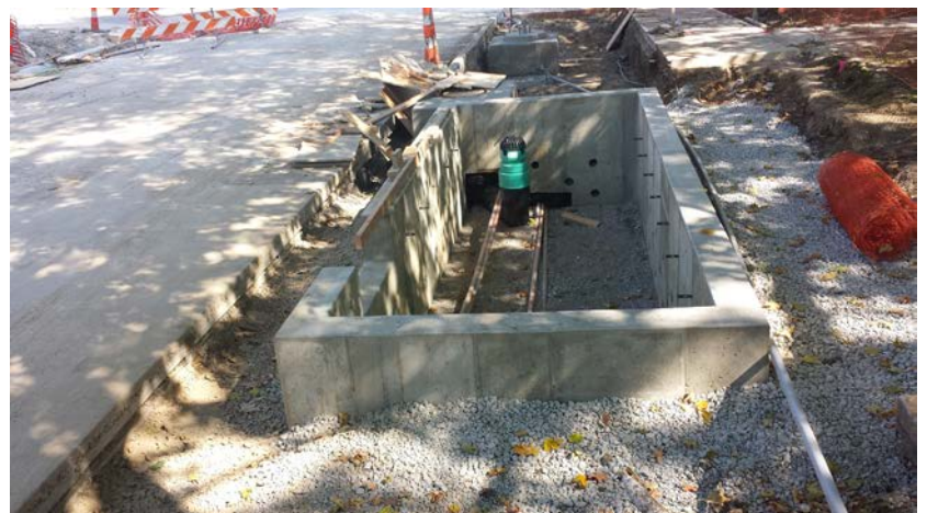
Planter box construction in Coralville.
