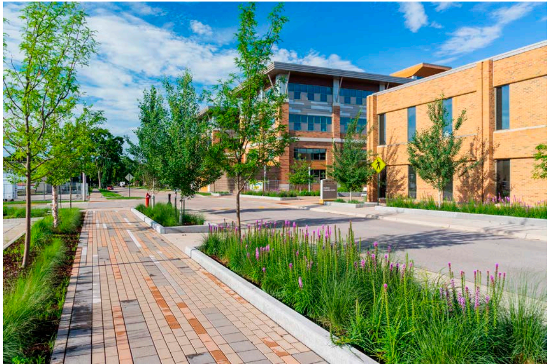
Stormwater planters in La Crosse, WI include native perennials and trees.
