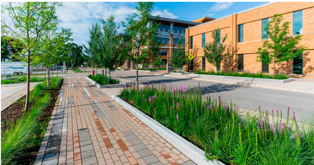
Stormwater planter boxes in La Crosse, Wisconsin.
