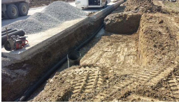
Photograph of a subdrain being installed in Coralville.
