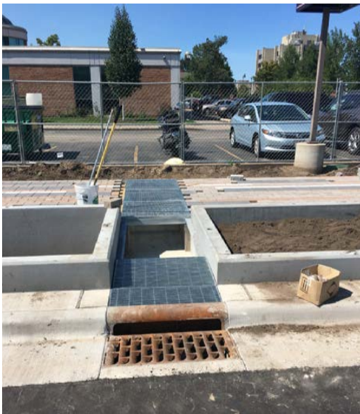
Installing grates over flume constructed in La Crosse, Wisconsin
