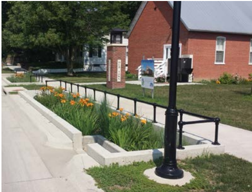
A cast in place concrete curb box is located downstream of the curb cut at the entry point to this planter box in Coralville.
