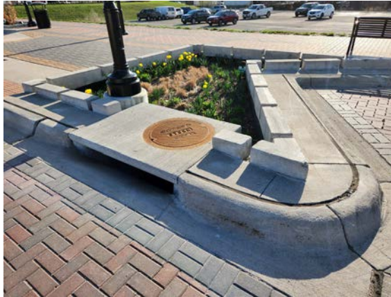
The level surface area within the planter box below the elevation of the adjacent street gutter is the ponding area at this location in Coralville.
