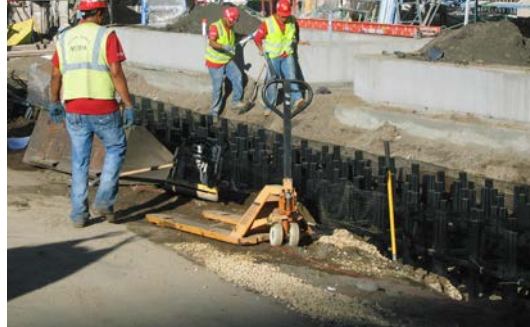
Structural cells under construction.
