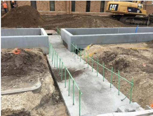
Cast in place flume construction in La Crosse, Wisconsin.
