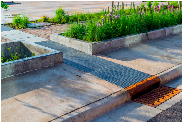
Catch basin sump installed in La Crosse, Wisconsin.
