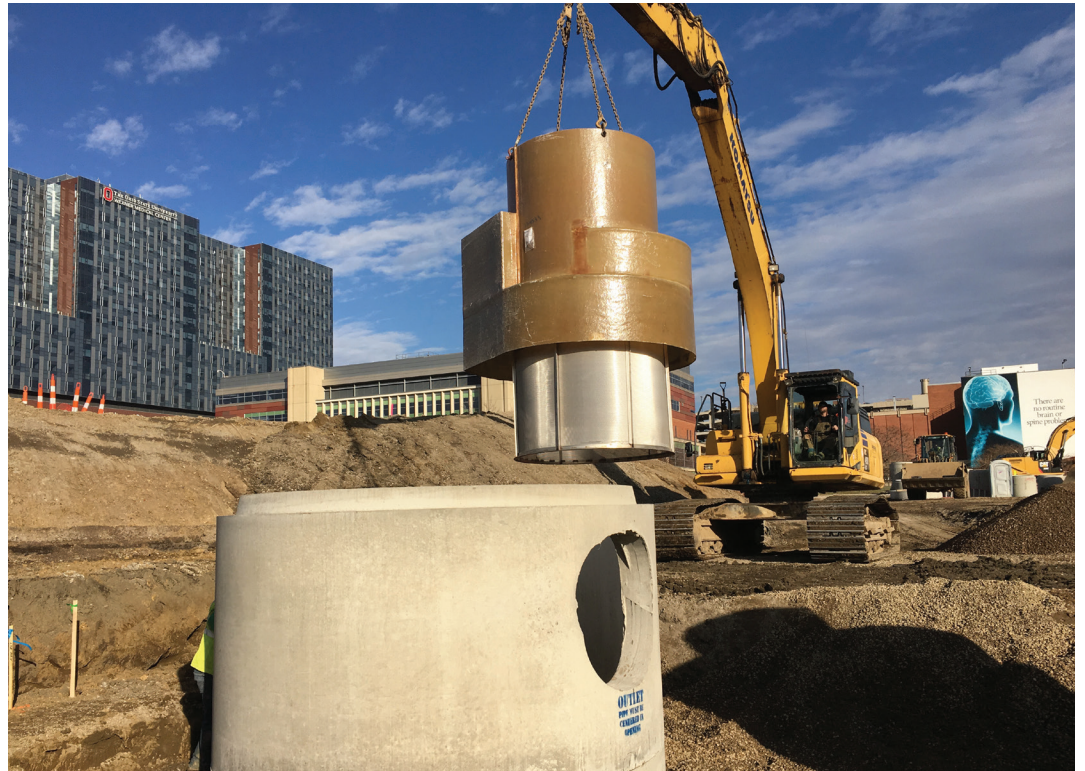
HDS system being installed.
