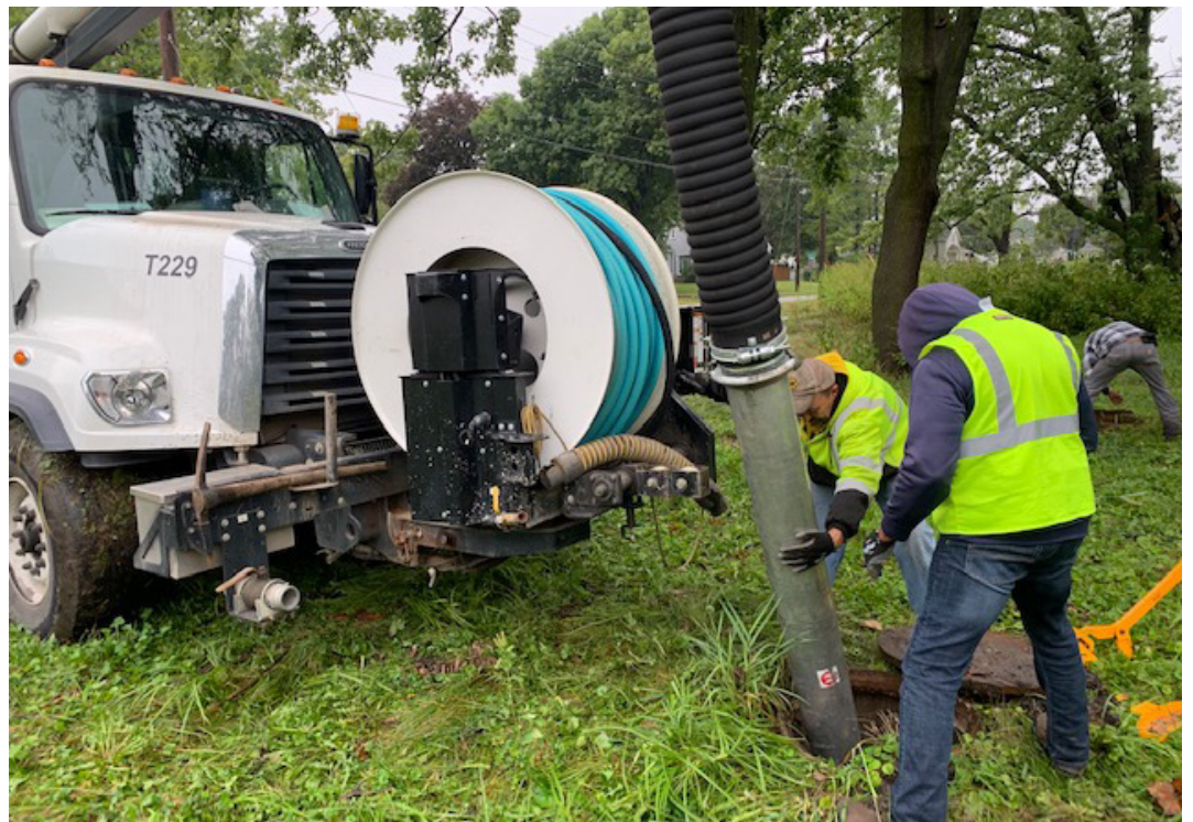
HDS device being maintained using a vacuum truck.
