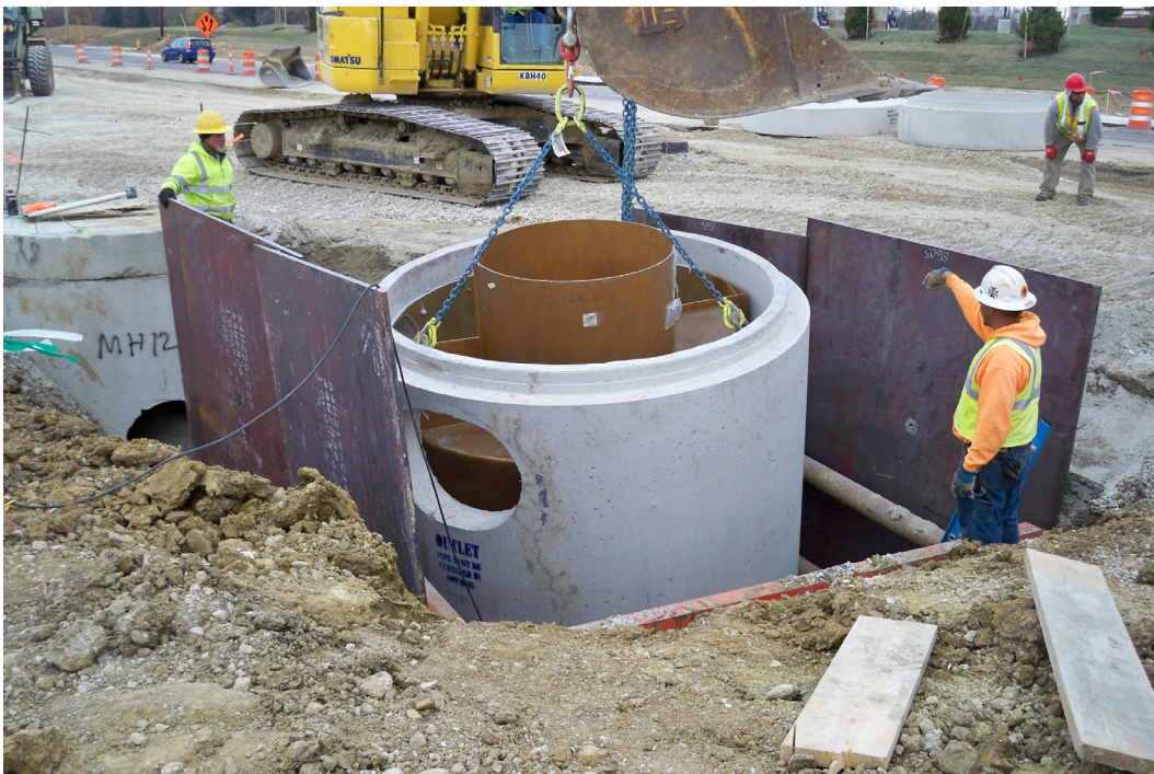
HDS system being installed.
