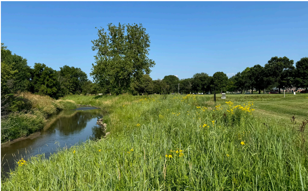
Vegetated Filter Strip along a creek in Davenport, Iowa.
