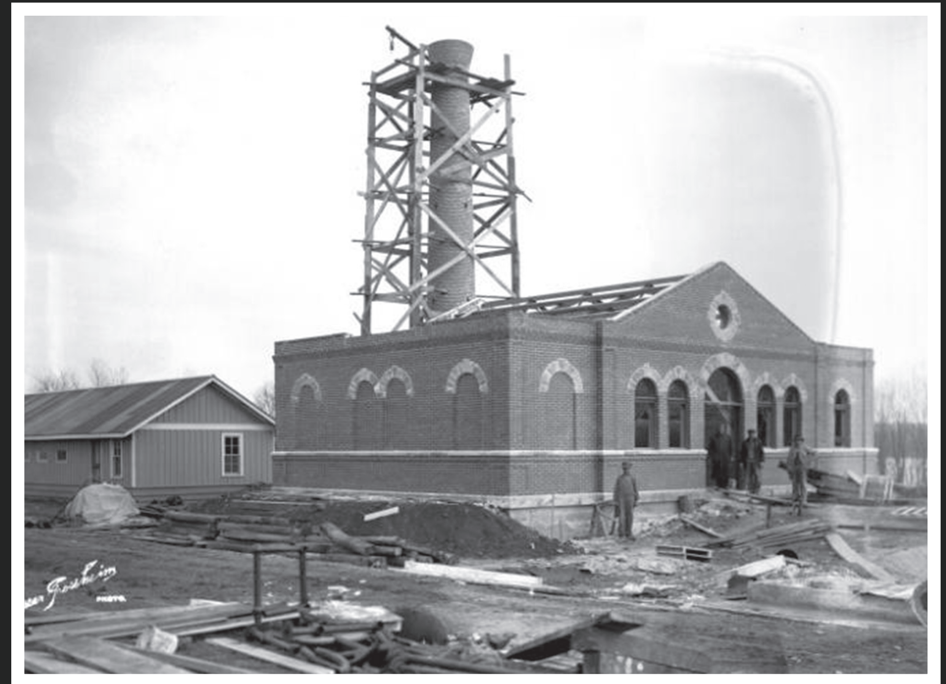
Overview of the Pumphouse during construction in 1910, facing southeast.
