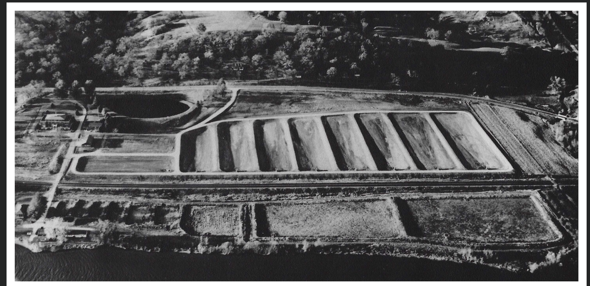
Aerial overview of hatchery showing new pond construction in mid-1950s, facing north.
