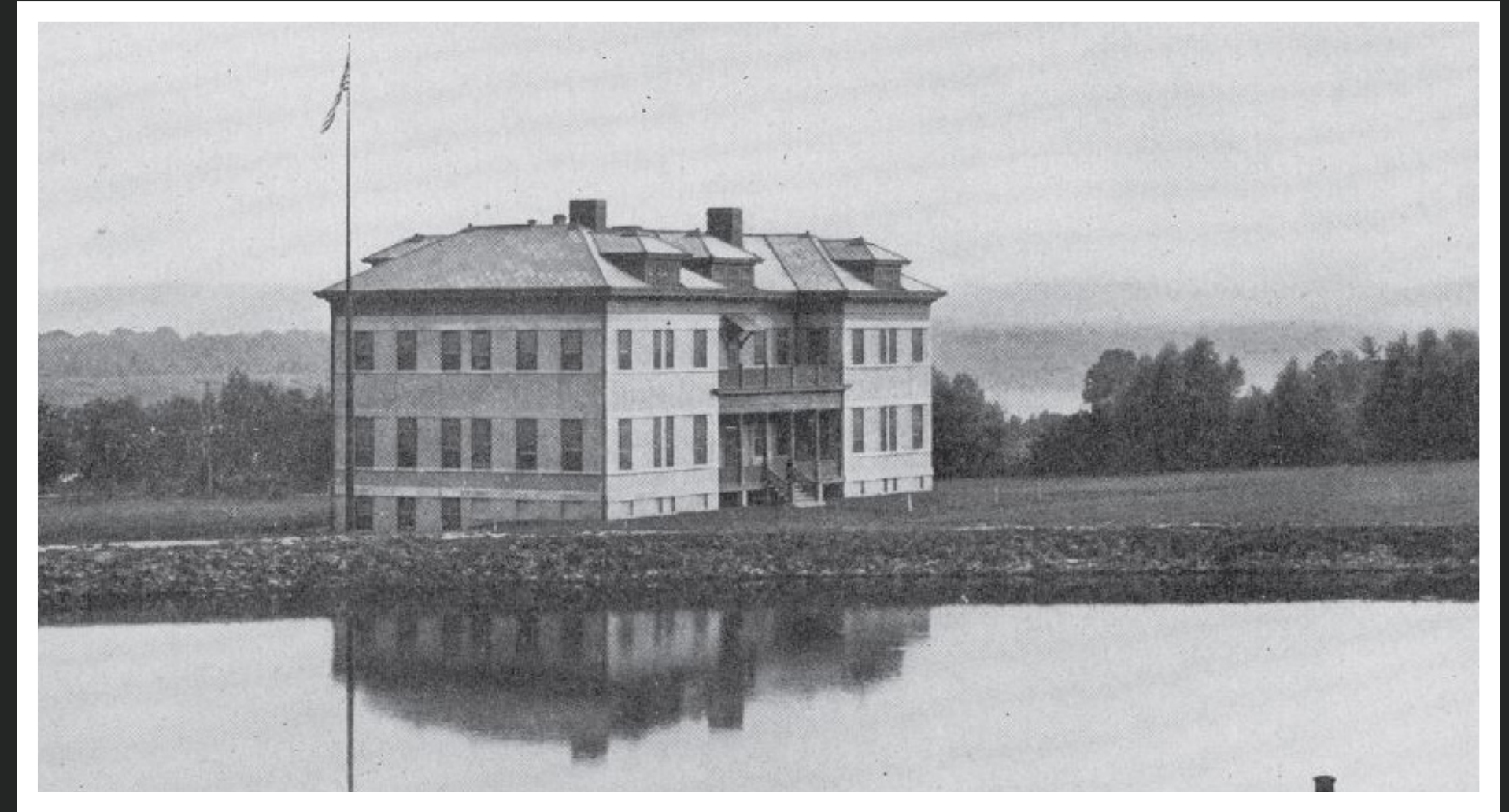
Overview of Main Laboratory circa 1914, facing southwest.
