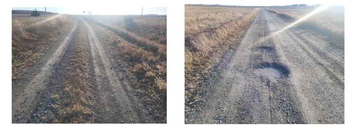
High vehicle traffic has worn the roadway crown down, which leads to standing/ponding water on the roadway, and resulting potholes. This project will repair all potholes, regrade the existing roadways to reestablish the roadway crown, and remove any high shoulder material (this will also help with roadway drainage). In addition, rock will be added to all roadways within this project area.
