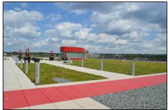
(b) A semi-intensive green roof at Cedar Rapids Public Library completed in 2013.
