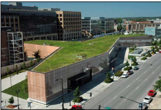
(a) An extensive green roof installed on the 70,000 square foot roof of the Des Moines’ downtown library in 2005.
