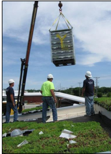
Figure C17-S1- 4: Installation of modular tray system green roof.
