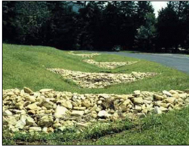
Figure C9-S2- 2: Grass swale with check dams (berms)
