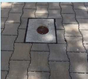
FIGURE C8-S1-12: Various types of observation wells
