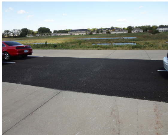
FIGURE C8-S1-5: Porous asphalt section in parking lot and closeup.
