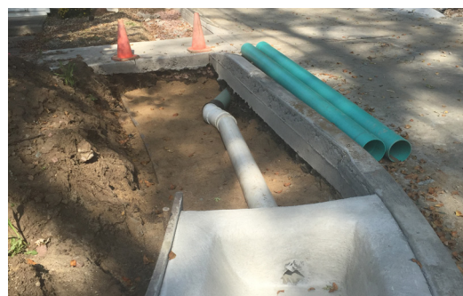
FIGURE C8-S2-5: Laying of underdrain systems
