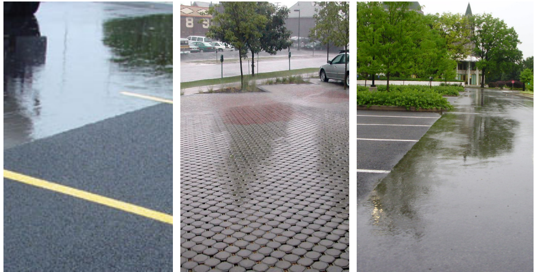
FIGURE C8-S1-8: Draining pervious areas adjacent to permeable pavement
