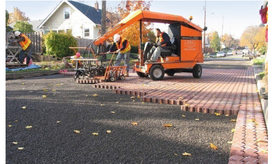
FIGURE C8-S2-7: Installing bedding and pavement courses
