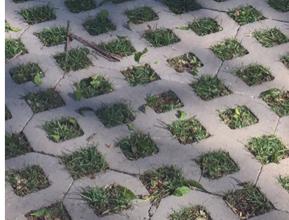
FIGURE C8-S1-3 Open Void Pavers example.
