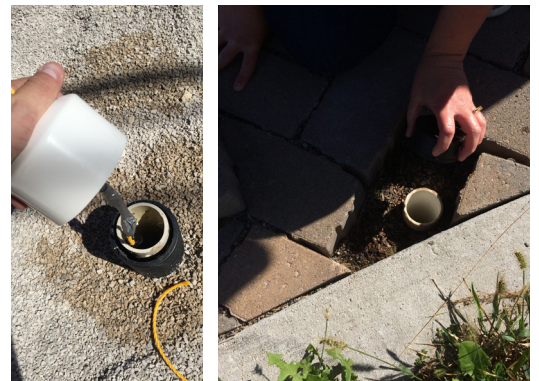
FIGURE C8-S1-13: Installation of observation wells and clean-out
