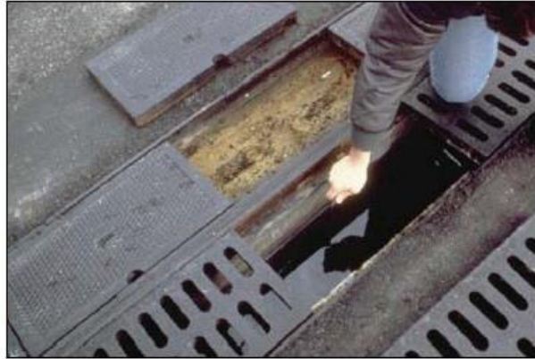
Figure C6-S1- 6: Perimeter sand filter
