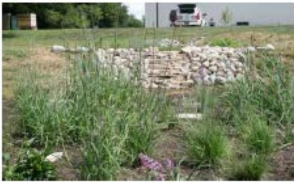
(a) Cascading feature in two-stage bioretention cell.
