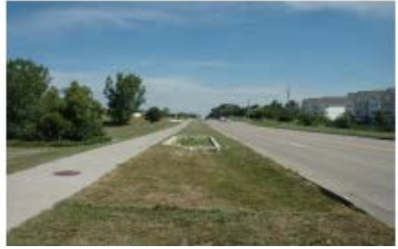
(b) The grassed pretreatment area provides a long flow path to this bioretention cell. Curb cuts were installed after the young plants became established.
