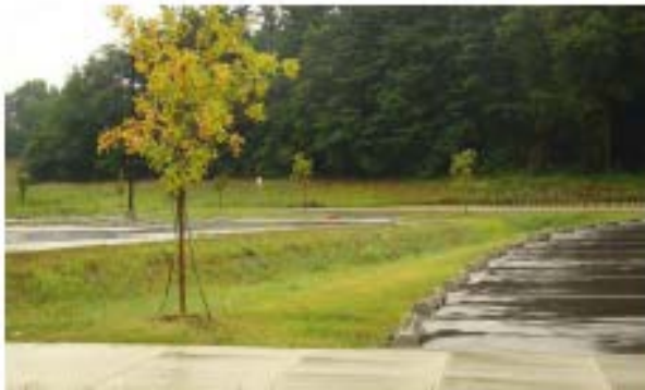
(c) Newly planted bioretention area with native grasses
