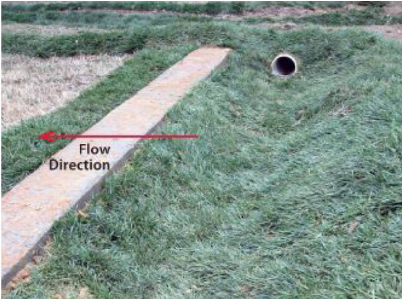
Concrete level spreader with grass basin on upstream side. Flow enters from pipe that runs parallel to the spreader and leaves by filling the basin and flowing across the level concrete strip. (photo courtesy - NC State University "Urban Waterways - Level Spreader Update")
