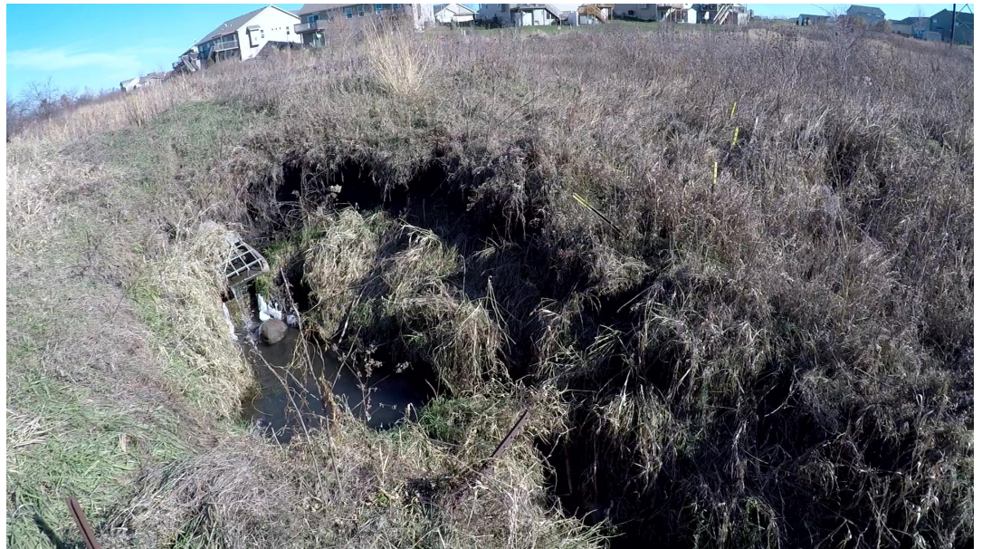
Figure 9.09-1-11: Unstable outfall
