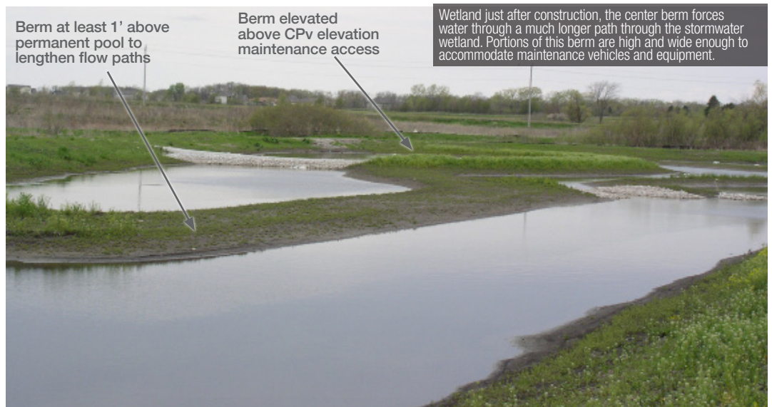
FIGURE 9.08-1-10: TOPOGRAPHIC ZONES WITHIN A STORMWATER WETLAND
