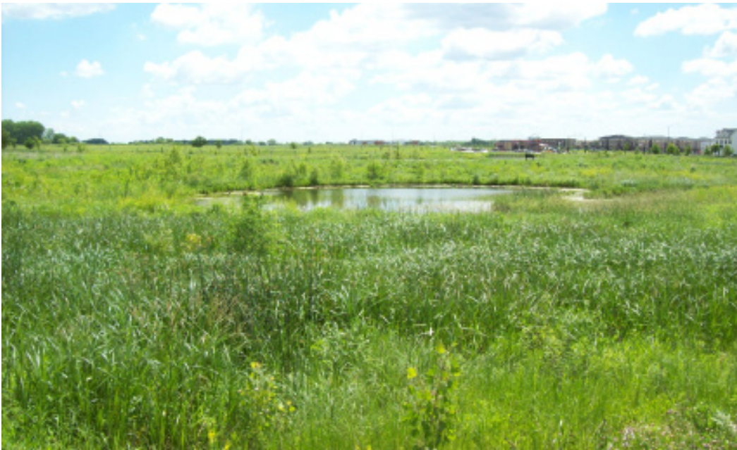
Established stormwater wetland in Prairie Trail, Ankeny, Iowa
