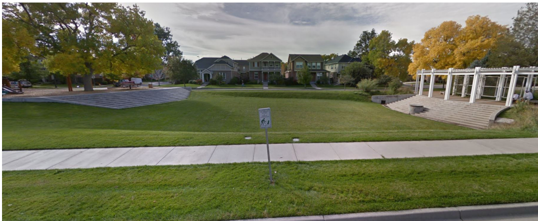
Photo 9.01-3-2: Example of passive detention at Sunset Park in Denver, Colorado (photo credit Google Maps)
