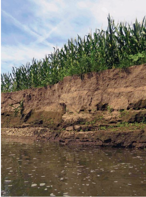
Scoured river bank
