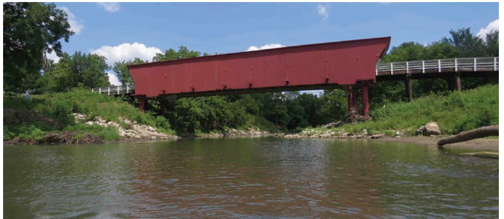
Side view of Roseman covered bridge
