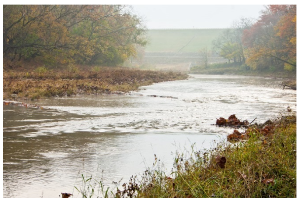
Photo 14. Stillwater River post-restoration in Englewood, OH following dam removal. Source: Stantec.
