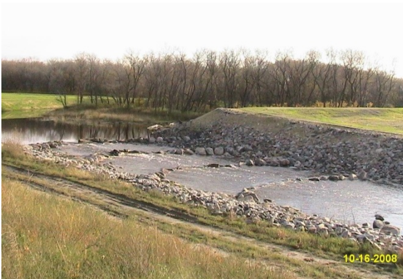
Photo 15. Example of rock ramp structure for fish passage and grade control. Source: Unknown.
