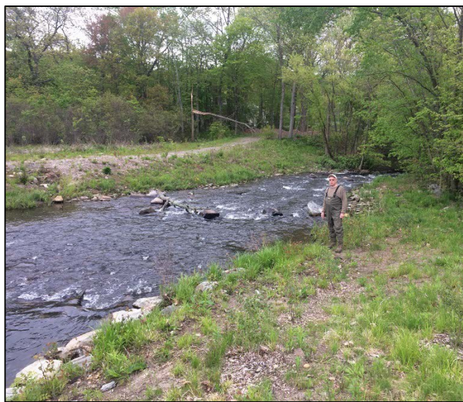
Photo 18. Pond Lily Dam location following replacement of dam function with free-standing fish-passable grade control. Source: Stantec.
