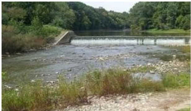
Photo 11. Englewood Dam in Englewood, OH prior to phased removal. Source: Stantec.
