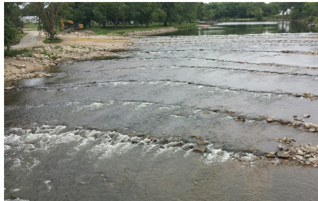
Photo 16. Rock arch rapid following Quasqueton Dam removal. Source: Iowa DNR.
