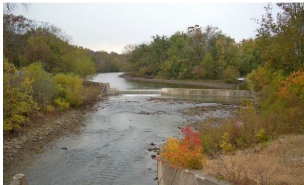
Photo 12. First stage of dam removal at Englewood Dam. Source: Stantec.
