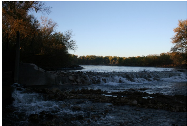
Photo 10. Coggon dam after 1 st stage of dam removal. Source: Iowa DNR.
