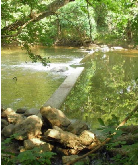
Photo 1. Low-head dam on Deer Creek in Williamsport, Ohio. Source: Stantec.
