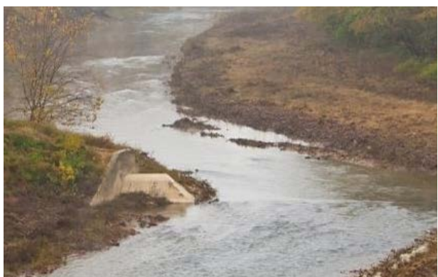
Photo 13. Further stage of dam removal in Englewood, OH. Source: Stantec.
