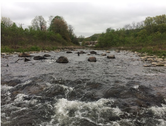
Photo 19. View of free-standing fish-passable grade control at Pond Lily Dam site. Source: Stantec.
