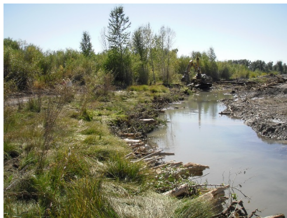
Photo 4. Toe wood installation during construction. Source: Wildland Hydrology.
