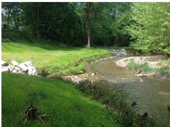
Photo 7. Finished bank with stone toe protection following revegetation. Source: Stantec.
