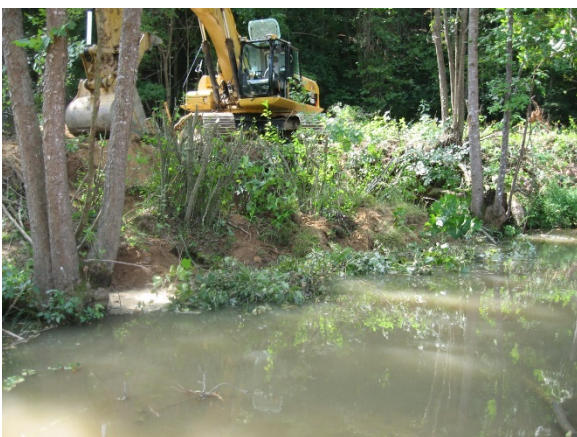
Photo 1. Toe wood with sod mats. Source: Wildland Hydrology.
