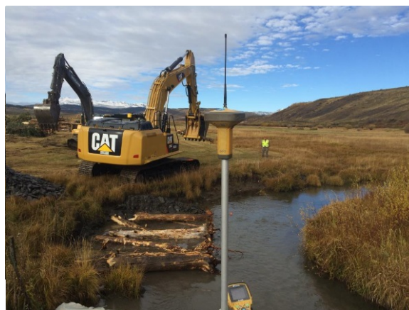
Photo 2. Installation of toe wood protection. Source: Stantec.
