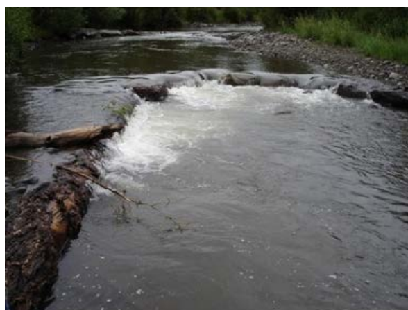
Photo 15. Log vane with boulder hook on Ohio Creek. Source: NRCS.
