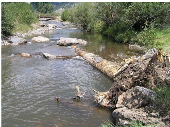
Photo 12. Log vane with boulder hook. Source: Stantec.
