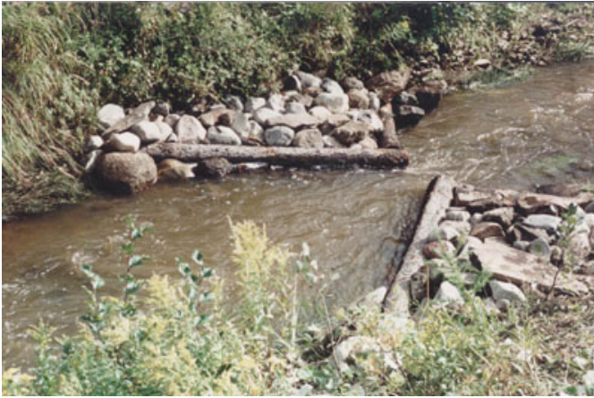
Photo 16. Double wing deflector. Source: corduroybrook.org .
