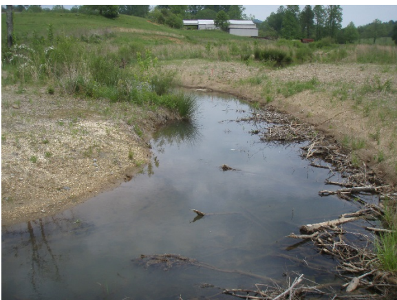
Photo 3. Newly constructed toe wood protection. Source: Stantec.
