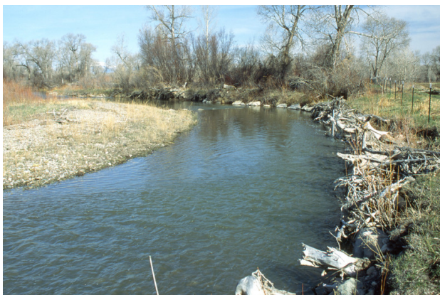
Photo 9. Root Wad channel bank protection. Source: NRCS.
