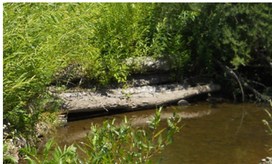
Photo 2. Installed LUNKER structure. Source: Dave Derrick, 2013.
