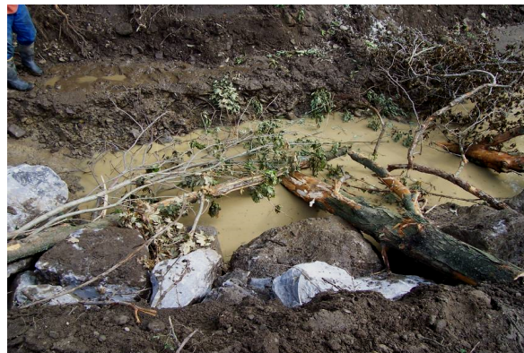
Photo 6. Locked Log structure during construction. Source: Dave Derrick, 2013.
