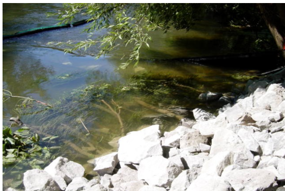
Photo 5. Constructed Locked Log structure. Source: Dave Derrick, 2013.
