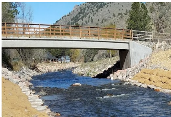
Photo 3. Boulder Cluster downstream of bridge. Source: Stantec
