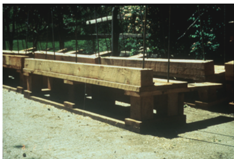
Photo 1. Constructed LUNKER structure. Source: Dave Derrick, 2013.
