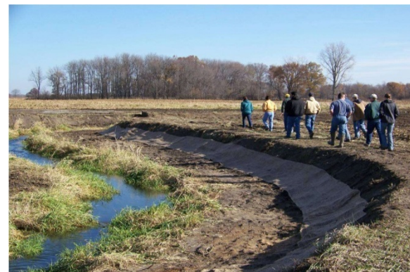
Photo 12. Bankfull benches after construction. Source: The Nature Conservancy
