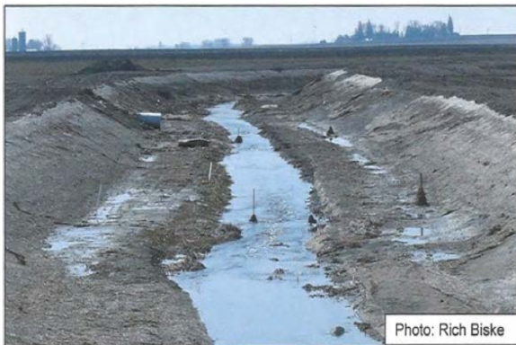
Photo 14. Example 2 - Two-stage channel during construction. Source: The Nature Conservancy
