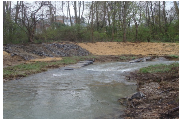
Photo 10. Big Cove Creek after bench construction. Source: Fulton County Conservation District
