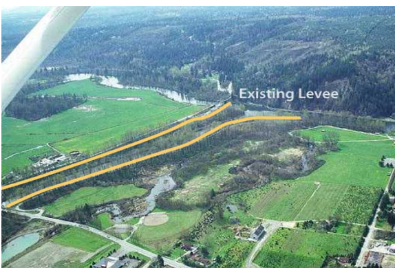
Photo 21. Levee location prior to relocation. Source: King County, WA
