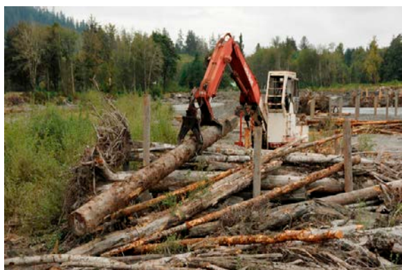
Photo 15. Floodplain assemblage structure during construction. Source: The Nature Conservancy
