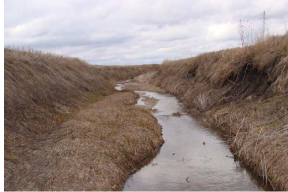
Photo 24. Example 1 – Post construction 2-stage channel. Source: University of Minnesota
