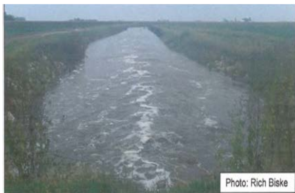
Photo 27. Example 2 - Two-stage channel during a flood event. Source: The Nature Conservancy
