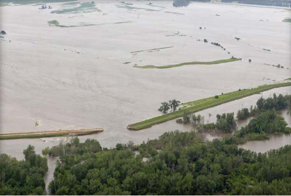
Photo 17. Levee breach near Hamberg, Iowa. Source: CBS News
