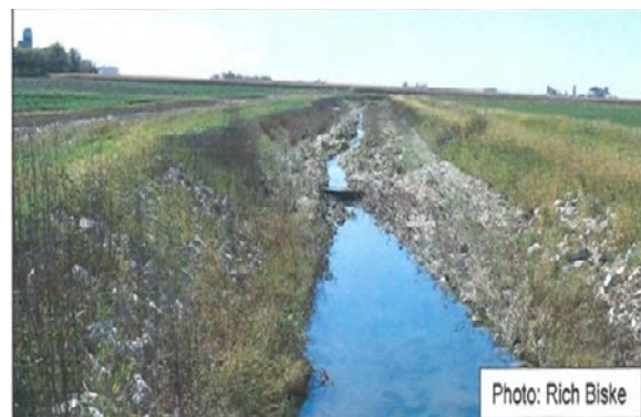
Photo 28. Example 2 - Two-stage channel after vegetative establishment. Source: The Nature Conservancy
