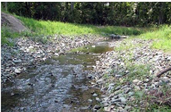
Photo 5. Example 2 - Reshaped stream bank after vegetative growth. Source: The Nature Conservancy & City of Charlottesville
