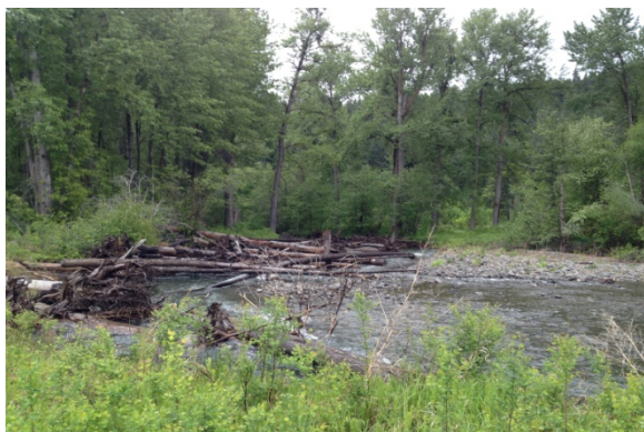
Photo 13. Large woody debris placement for floodplain restoration. Source: North West Fisheries Science Center
