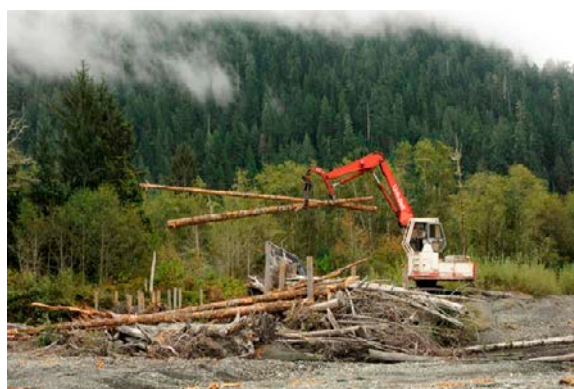
Photo 14. Floodplain assemblage structure during construction. Source: The Nature Conservancy
