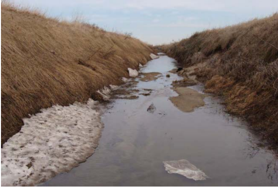
Photo 23. Example 1 – Pre-construction aggrading channel with trapezoidal geometry. Source: University of Minnesota
