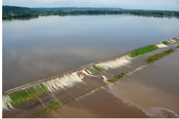
Photo 18. Levee overtopping. Source: USACE
