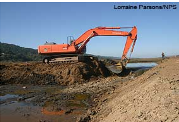
Photo 19. Levee removal. Source: National Park Service
