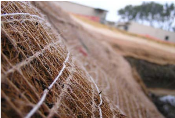
Photo 28. Erosion control matting. Source: Salix Applied Earthcare
