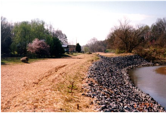
Photo 7. Joint planting. Source: Charlotte-Mecklenburg Storm Water Services
