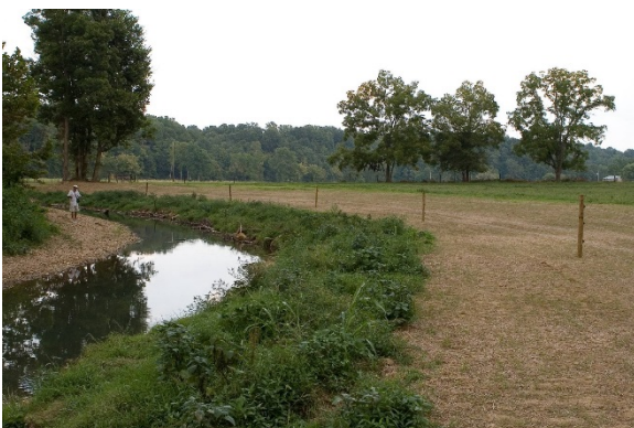
Photo 35. Sod matting on stream banks. Source: Stantec
