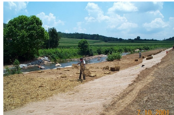
Photo 40. Apply mulch to seeded stream banks. Source: Buck Engineering
