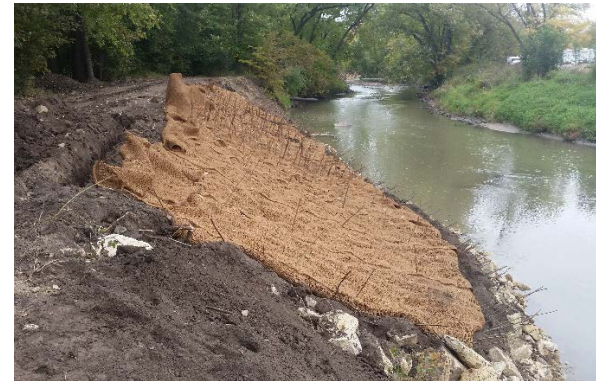
Photo 29. Erosion control matting installed on slope. Source: Iowa DNR
