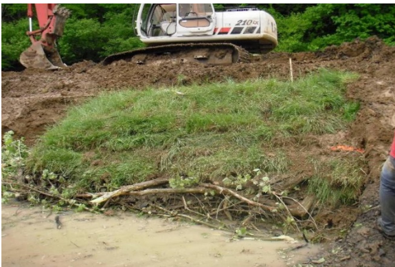
Photo 33. Sod mat stacked over toe wood. Source: Stantec
