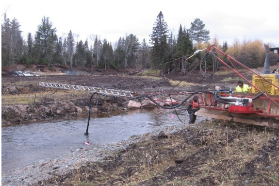
Photo 5. Hydraulic stinger live stake installation. Source: Lake Superior Tree Farm
