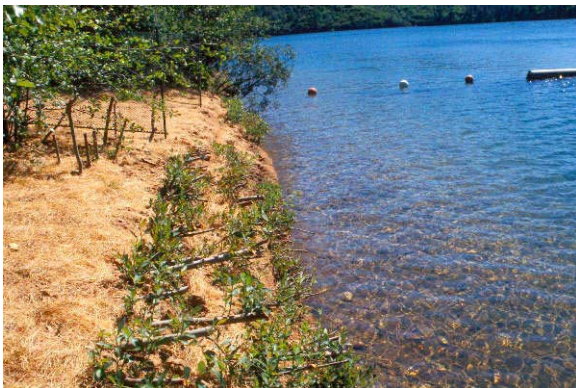
Photo 21. Brush layering, including soil wrap, Whiskeytown Lake, CA. Source: Salix Applied Earth Care
