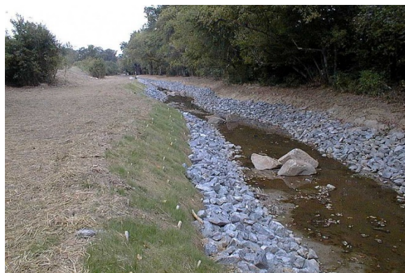
Photo 27. Erosion control matting with seed growing through. Source: Charlotte-Mecklenburg Storm Water Services
