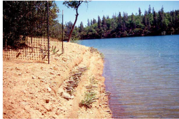
Photo 20. Brush layering, including soil wrap, Whiskeytown Lake, CA. Source: Salix Applied Earth Care
