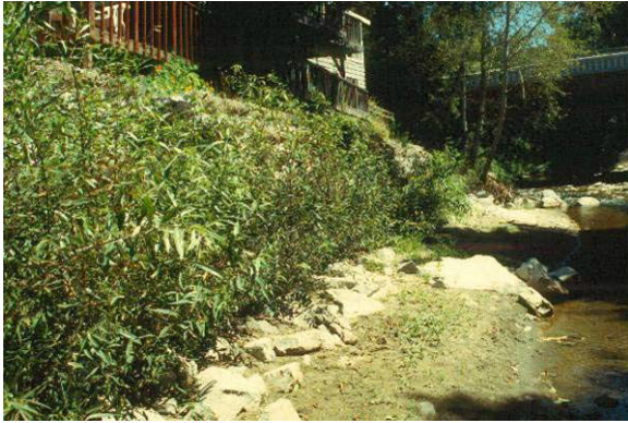
Photo 19. Brush Layering with soil wrap used to stabilize a stream bank. Source: Salix Applied Earth Care
