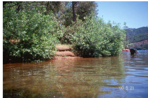
Photo 22. Brush layering, including soil wrap, Whiskeytown Lake, CA. Source: Salix Applied Earth Care
