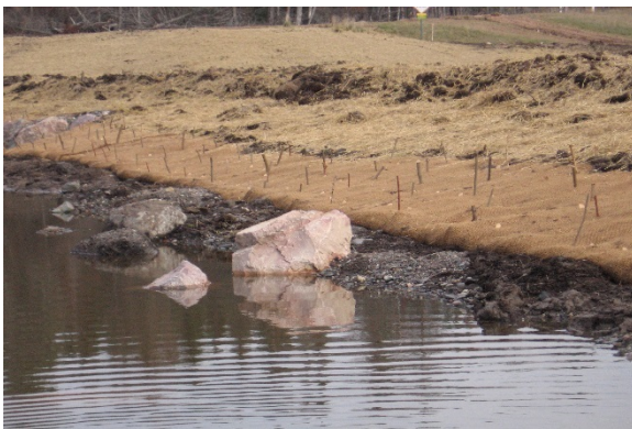
Photo 11. Live stakes in erosion control matting. Source: Collins & Baker Engineering
