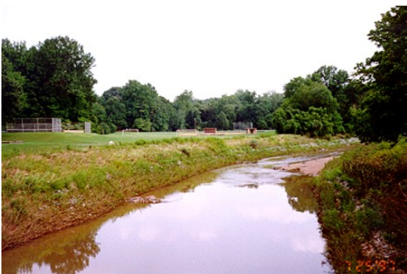
Photo 17. Fascines with new growth. Source: Charlotte-Mecklenburg Storm Water Services
