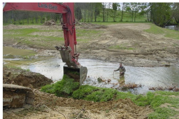
Photo 36. Excavator placing sod matting. Source: Bluegrass Streams, LLC
