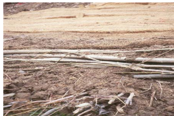
Photo 18. Installed fascine. Source: Stantec
