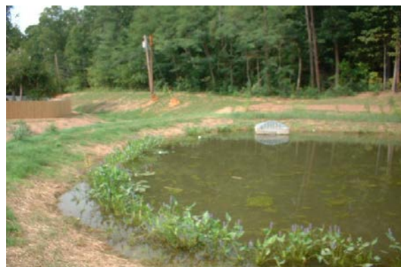
Photo 48. Vegetative plugs at Edwards Branch, NC. Source: Charlotte-Mecklenburg Storm Water Services
