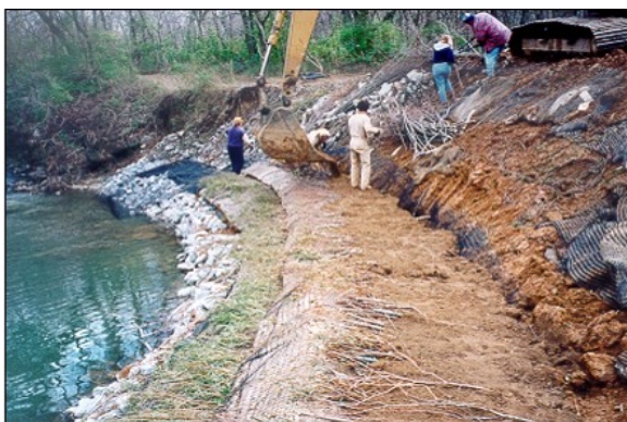
Photo 23. Bench excavation for brush layering. Source: Stantec
