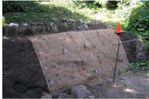
Photo 26. Erosion control matting installed on a slope. Source: Salix Applied Earthcare
