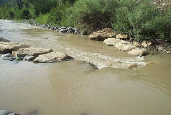
Photo 5. Cross vane on the Rio Blanco. Source: Wildland Hydrology.
