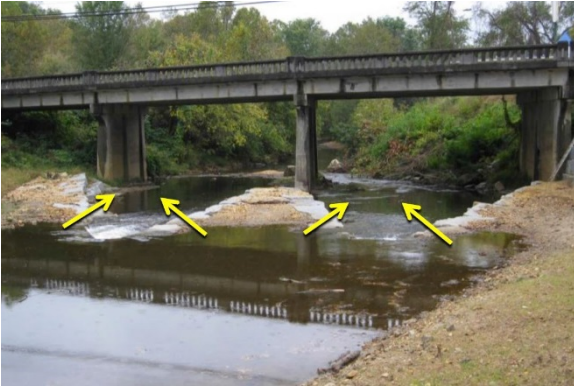
Photo 9. W-weir directing flow through bridge with center pier. Source: Unknown.
