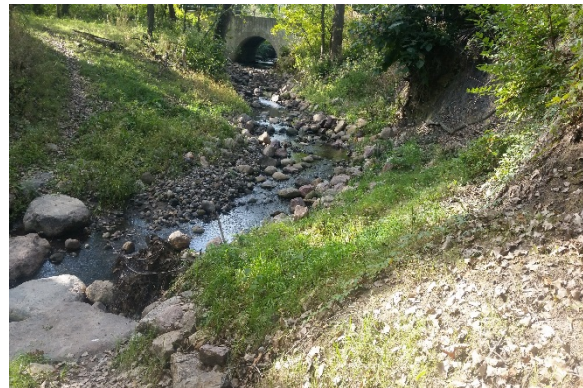
Photo 26. Rock constructed riffle at First Unitarian Church. Source: Iowa DNR.
