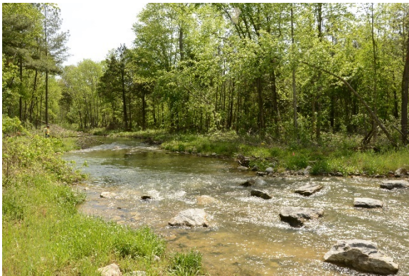
Photo 25. Rock constructed riffle with boulders dispersed throughout. Source: Stantec.
