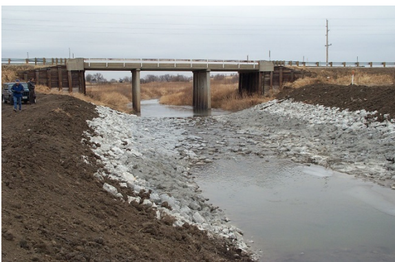
Photo 29. Grouted Grade Control Structure. Source: Hungry Canyons Alliance.
