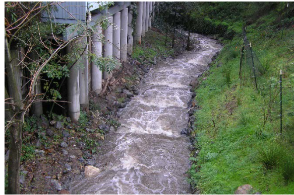
Photo 16. Step Pools along Codornices Creek. Source: Stantec.
