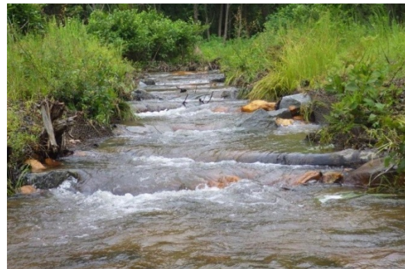
Photo 22. Rock and log riffle. Source: Wildland Hydrology.
