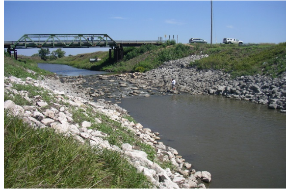
Photo 28. Grouted Grade Control Structure. Source: Hungry Canyons Alliance.
