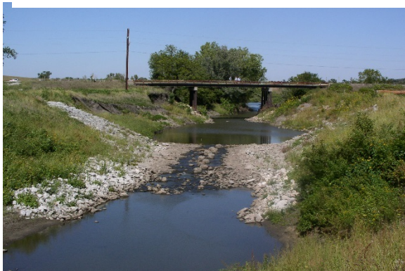
Photo 31. Grouted Grade Control Structure. Source: Hungry Canyons Alliance
