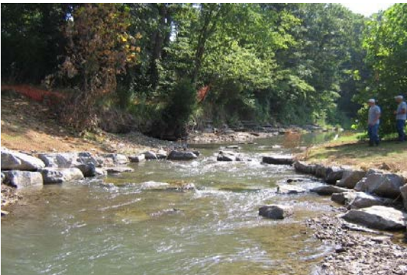
Photo 7. Cross vane with step. Source: Trammel Creek, Stantec.
