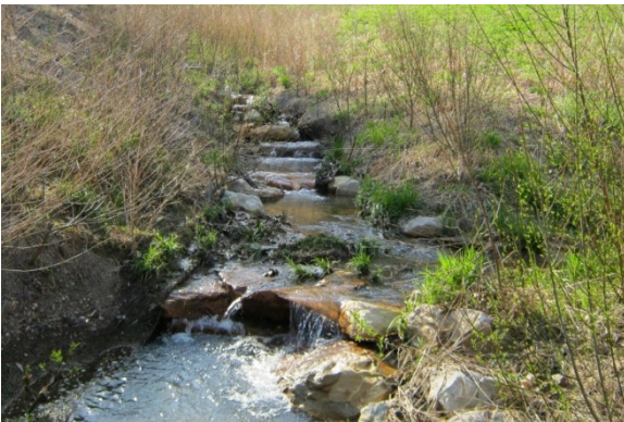
Photo 15. Boulder steps. Source: Stantec.
