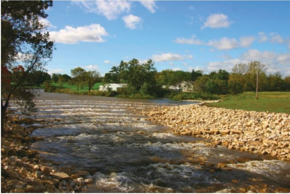
Photo 1. Rock Arch Rapids at Vernon Springs Dam site. Source: Howard County, IA, Economic Development.
