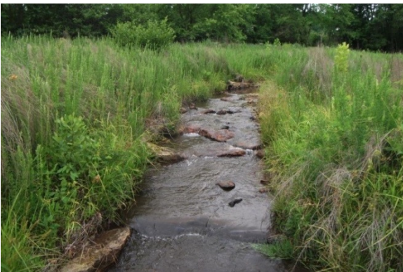
Photo 19. Rock and log riffle. Source: Stantec.
