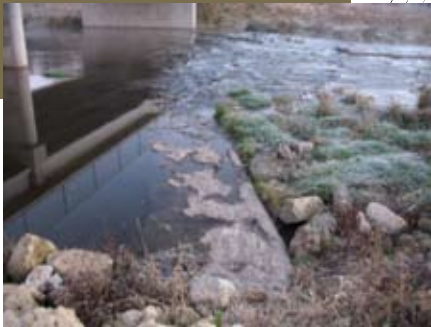
Height reduced. The height of the Hopkinton Dam was reduced, with a riffle installed downstream, similar to the Figure 4-l.
