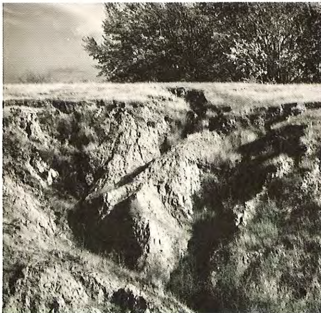
Gully erosion, Scott County Soil Conservation Service
