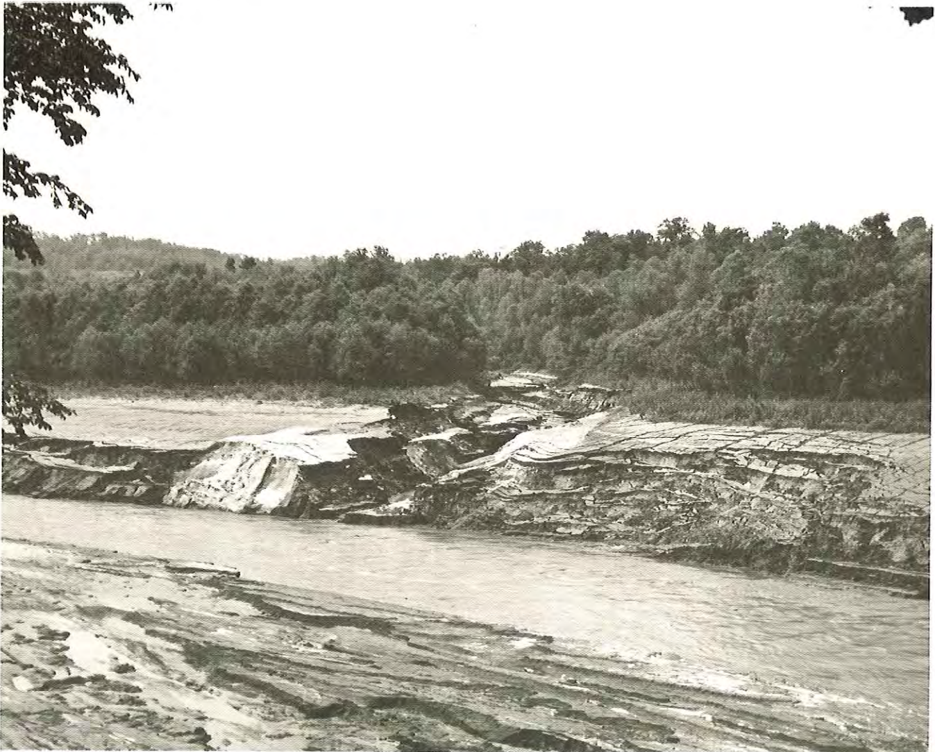
Silt accumulation upstream of Upper Iowa River Dam
