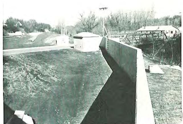
Floodwall along Mad Creek, Muscatine Corps of Engineers
