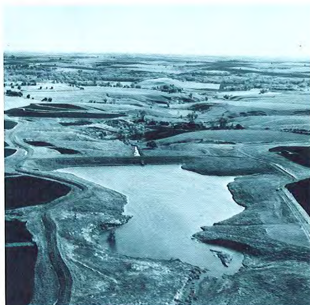
Watershed structure, Cherokee County Soil Conservation Service
