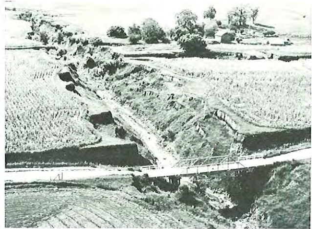
A gully in Woodbury County before treatment Soil Conservation Service
