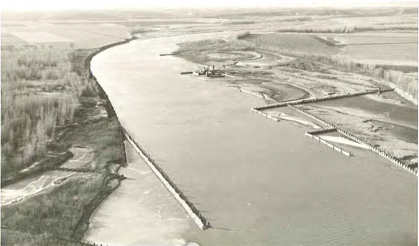
Channel stabilization on the Missouri River
