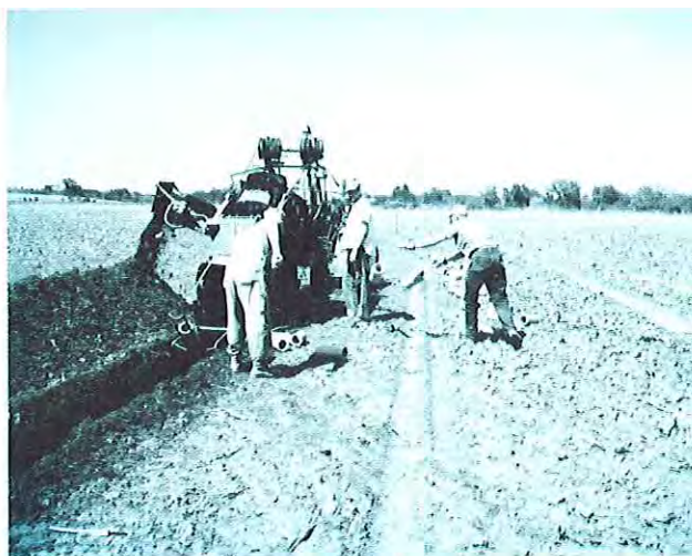
Laying tile to drain agricultural land Soil Conservation Commission
