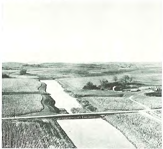
The same gully after treatment Soil Conservation Service
