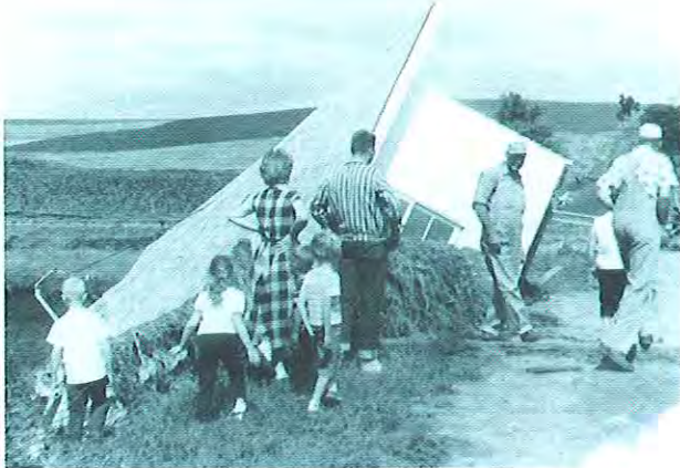
Flash flood damage at Audubon, July, 1958 Soil Conservation Service
