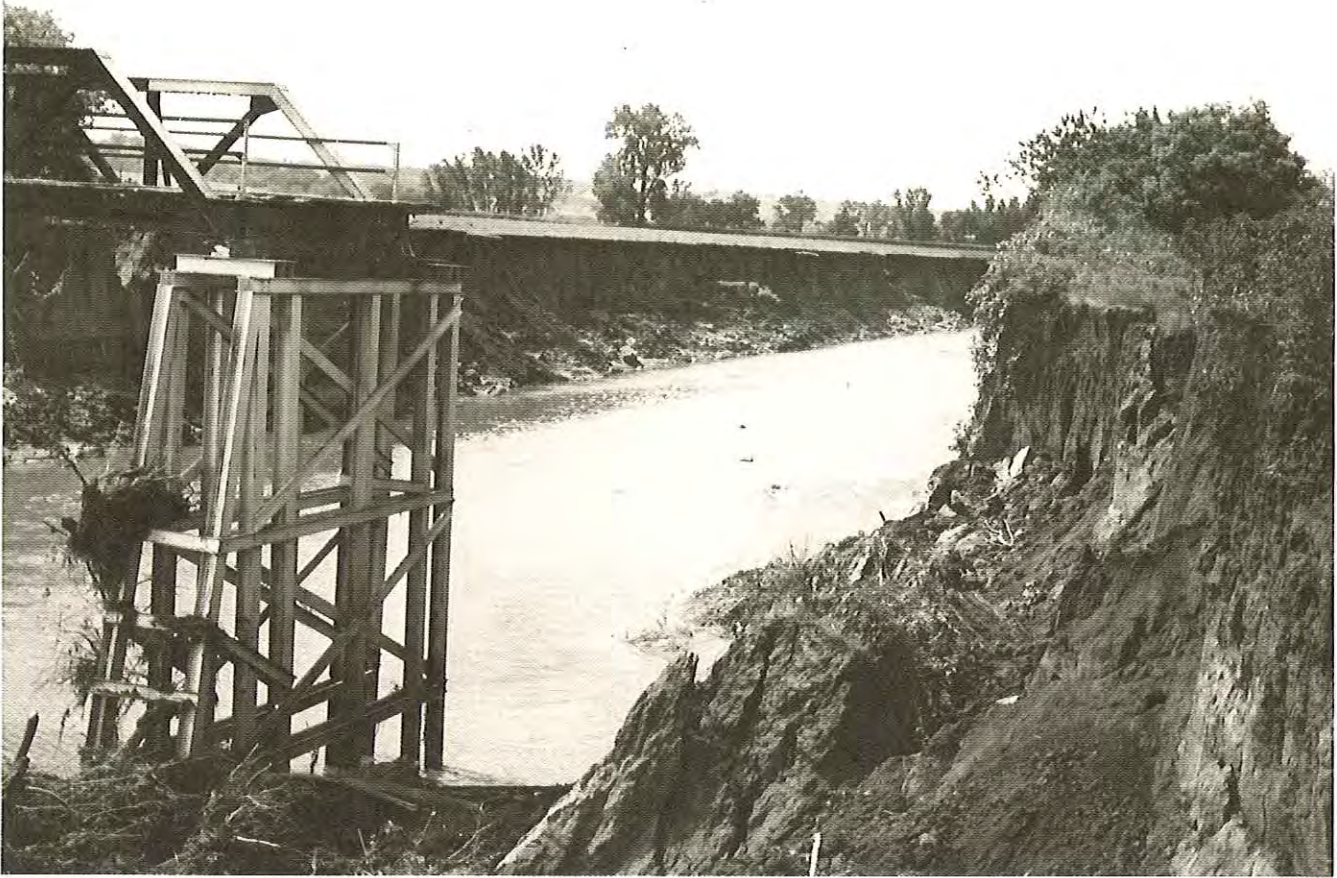
Streambank erosion on Soldier River, Monona County, 1950
