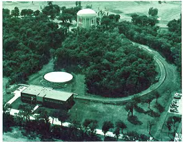
Municipal water supply, Fort Dodge City of Fort Dodge
