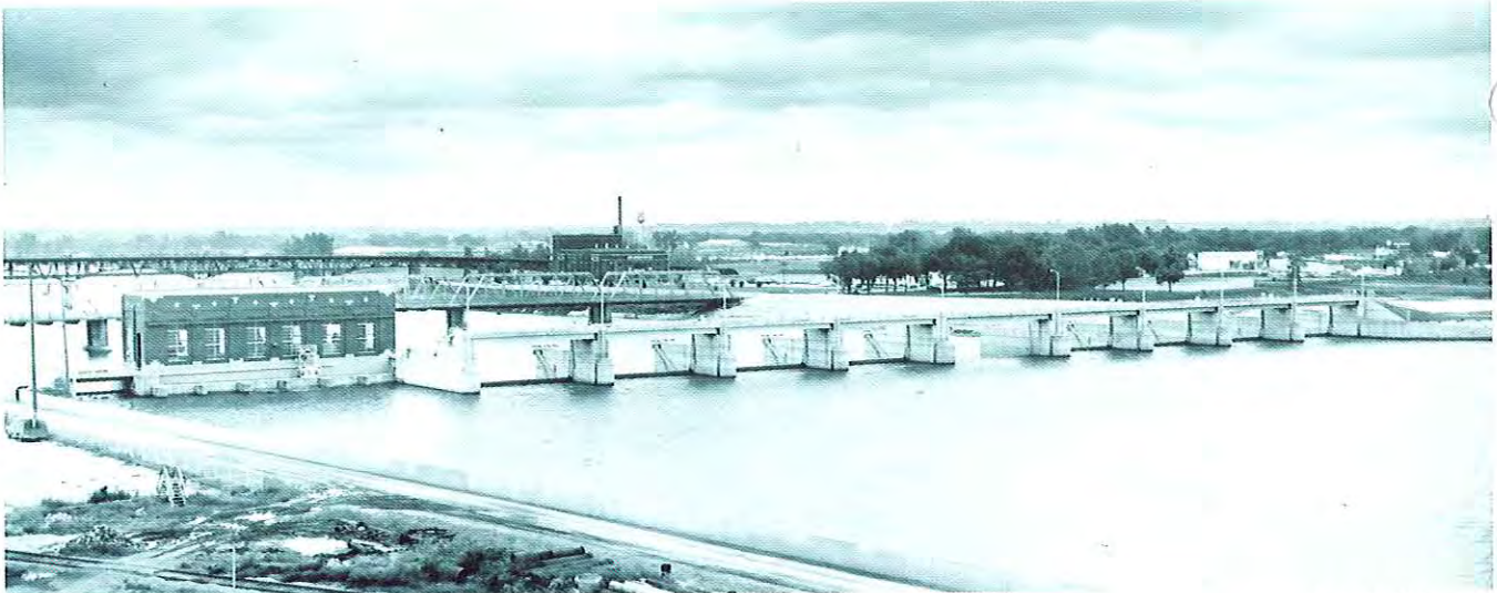
Hydroelectric power plant and dam, Ottumwa
