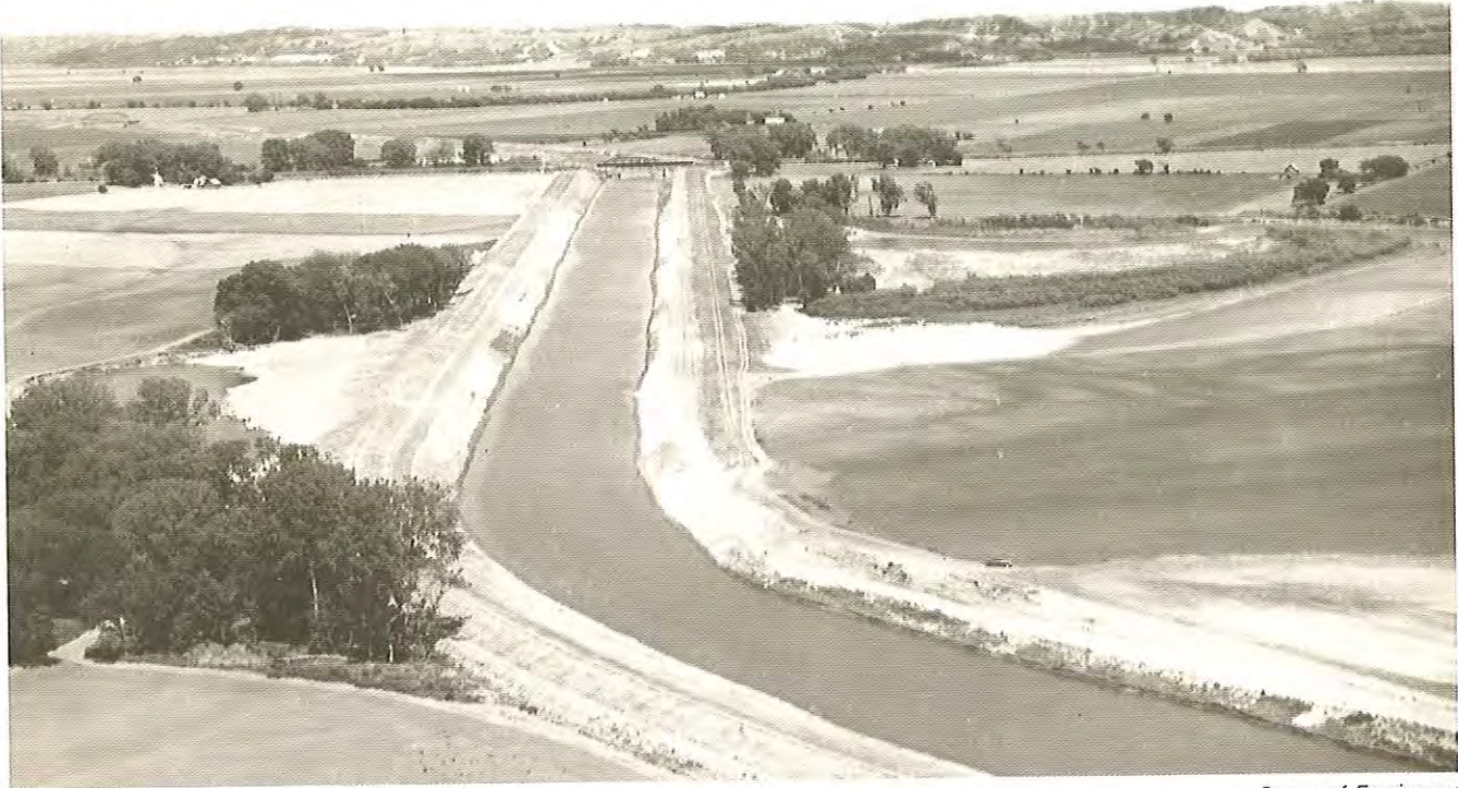
Channelization of Little Sioux River, Harrison County
