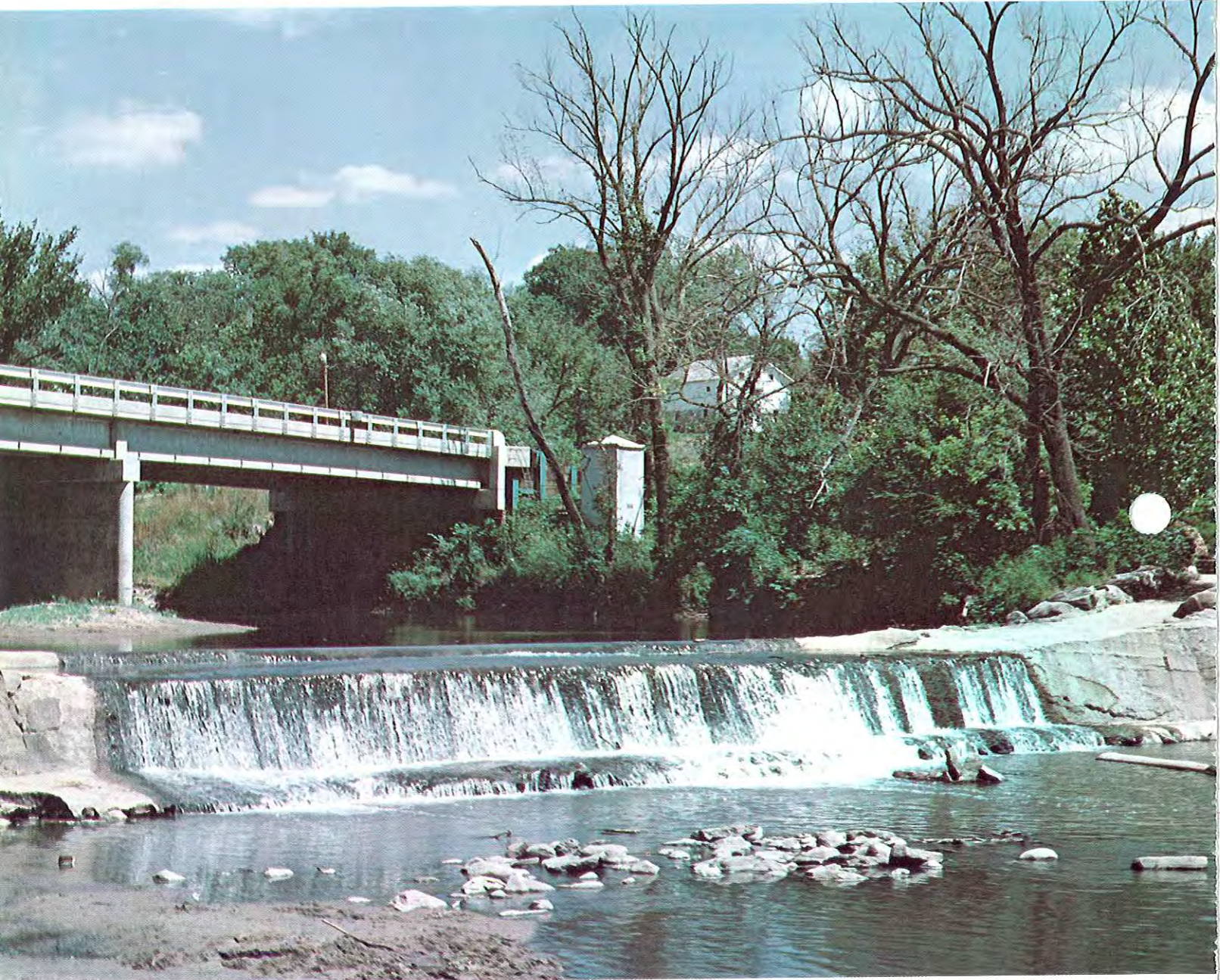
Stream gaging station on Raccoon River at Panora
