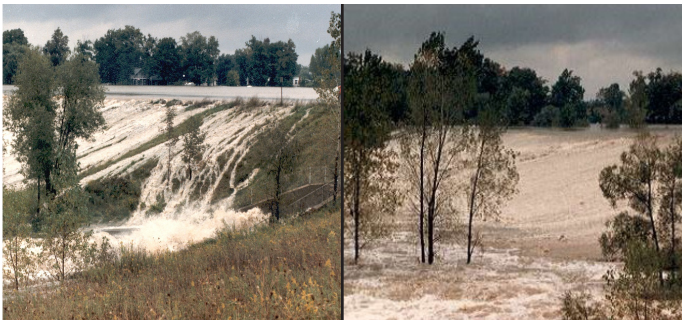
Figure 4: Examples of Dam Overtopping During a Flood
