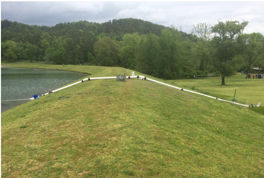
Figure 13: Example of Siphon System Installed on Embankment Dam
