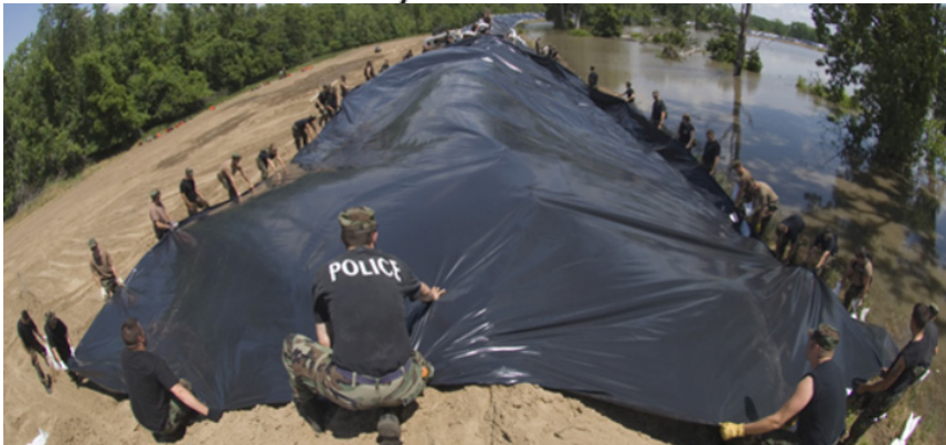
Source: USACE. Levee Owner's Manual for Non-Federal Flood Control Works (2006). Photo Source: U.S. Air Force
