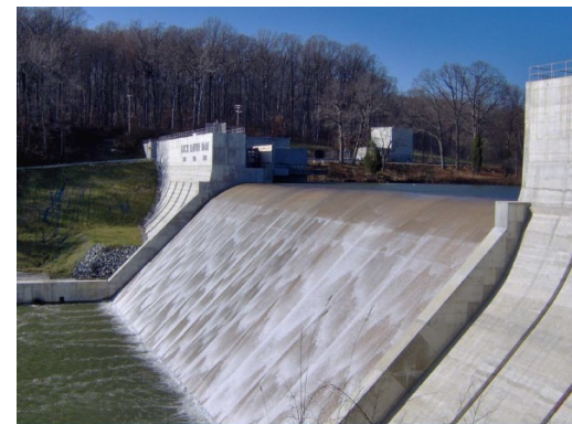
Selecting and Accommodating Inflow Design Floods for Dams
