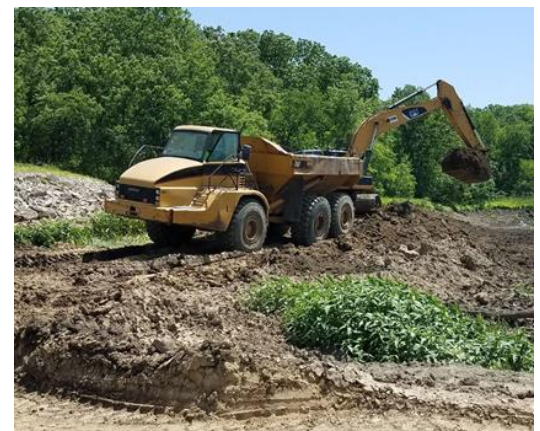
Construction equipment removes excess sediment from the lake bottom
