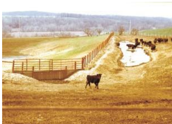
Solids settling structure with slotted gate.
