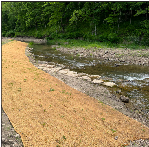
Rolled erosion control product used near a stream edge.
