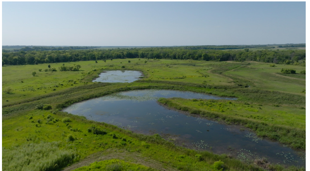
Constructed stormwater wetlands.
