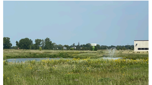
Wet detention pond.
