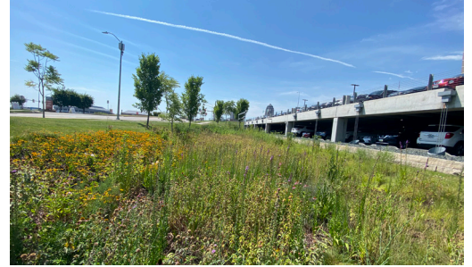
Dry detention basin.
