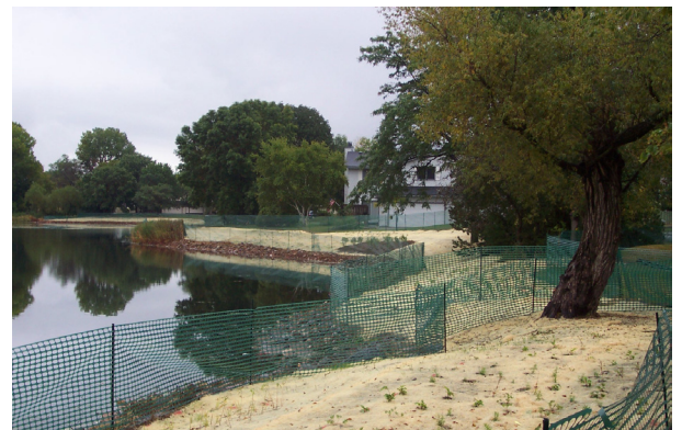
Fences used to protect vegetation from geese during construction.
