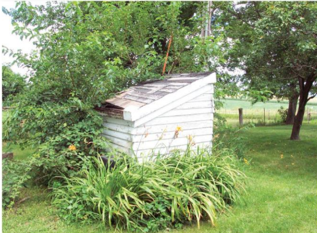
Examples of wells that should be plugged.
