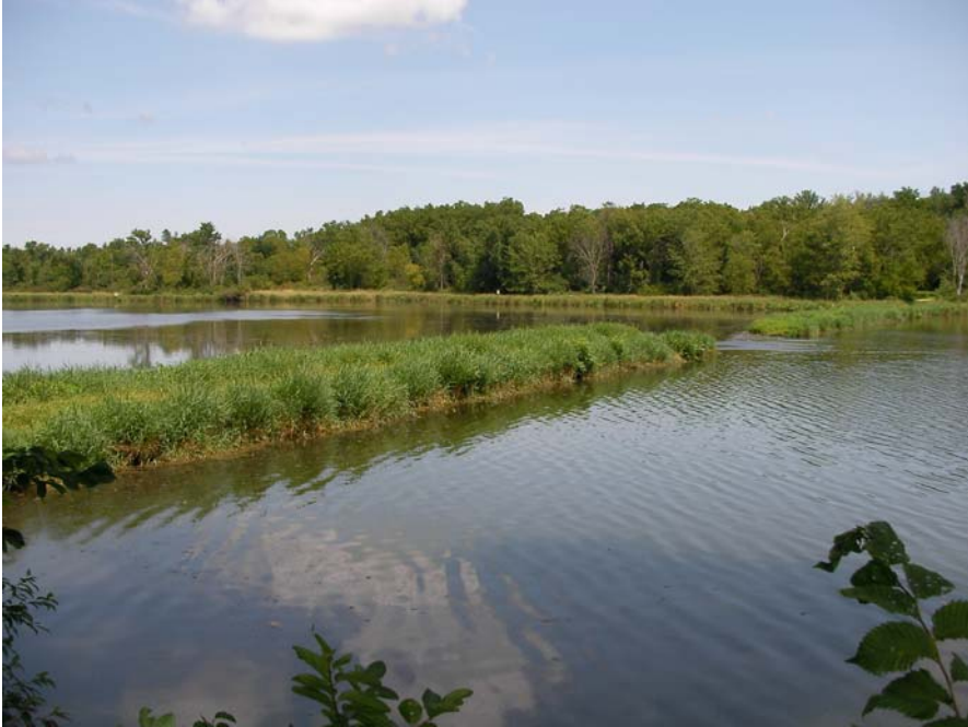
Figure D11 Union Grove Lake sediment control dike, looking east
