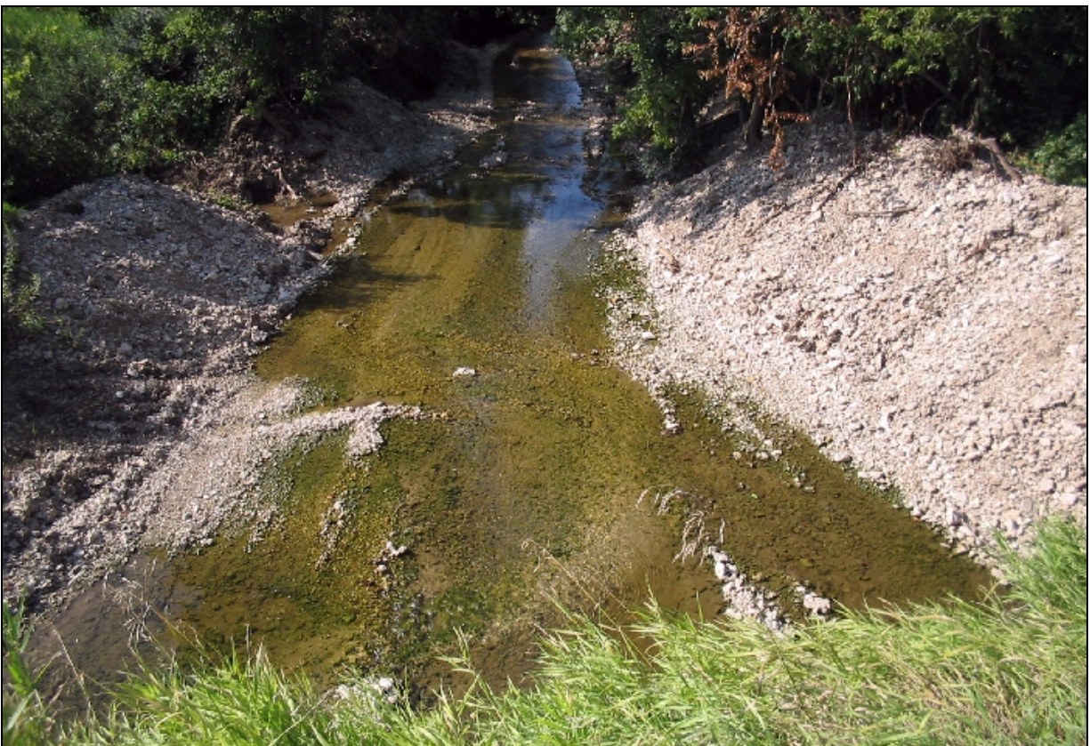
Figure 4-7. Hecker Creek at County Road W60 Bridge after Iowa DOT channel maintenance in 2004.
