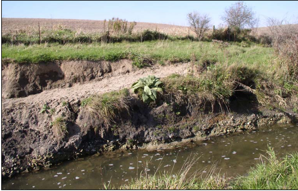
Figure 4-5. Bank erosion in Hecker Creek.
