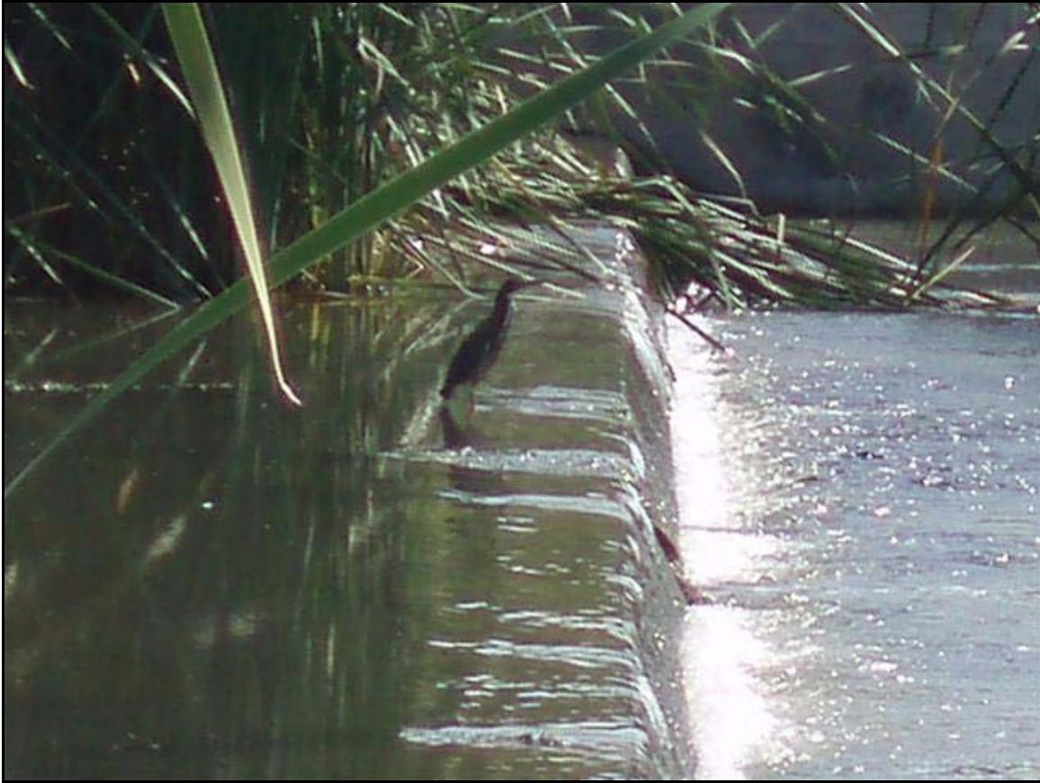
Figure 3. Low head dam separating Lower Gar Lake from Milford Creek (image from IDNR Use Attainability Analysis 2006).
