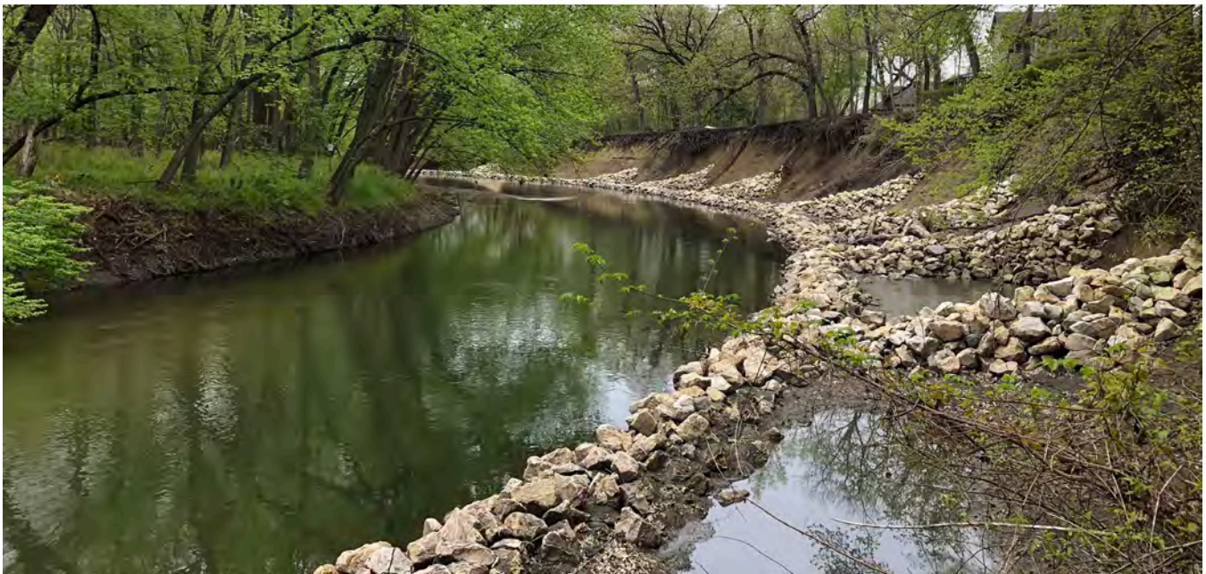
Bank stabilization project along Beaver Creek (City of Johnston).
