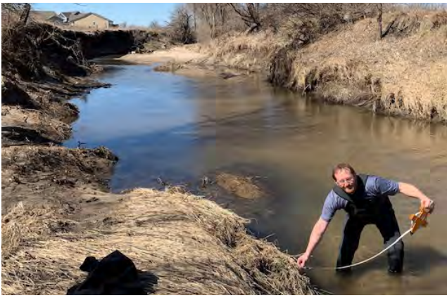
Monitoring conducted near an unstable stream bank (City of Johnston).
