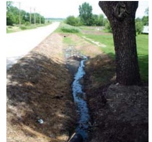
A failing septic system discharges sewage.
