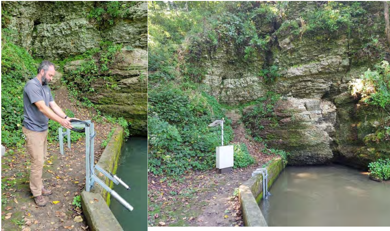
Figure 7. Water quality sensor installed at Siewers Spring to monitor water quality every 5 minutes. Data recorded from this sensor is available on the following website: https://iwqis.iowawis.org/app/ .
