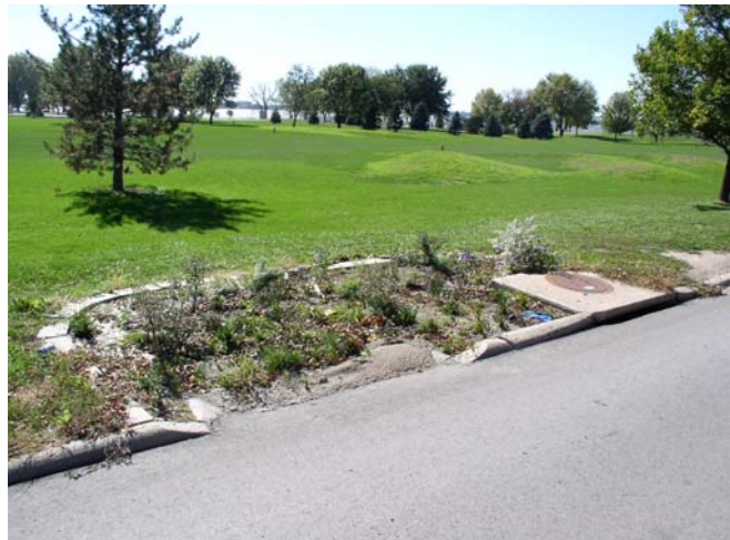
Example of a rain garden to capture runoff.
