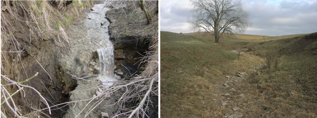
Left: One of at least 3 sinkholes in the Silver Creek stream corridor. Right: A dry segment of stream, downstream of the sinkholes.
