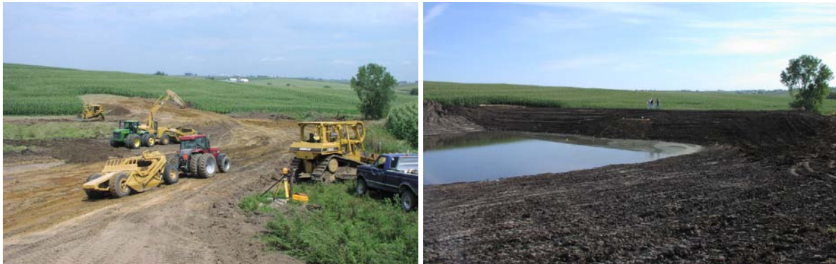
Construction and checkout of a new grade stabilization structure.
