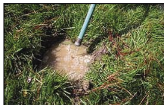
A percolation test should be conducted at any proposed rain garden site.
