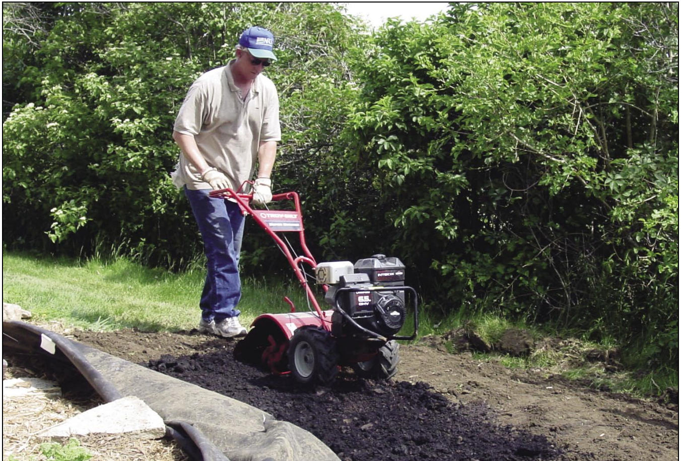
A rototiller is used to prepare a rain garden site in Madison County.
