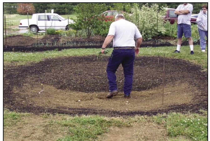
During this rain garden installation the area was over-excavated in sandy subsoil and backfilled with a soil amended with compost to increase organic matter content.
