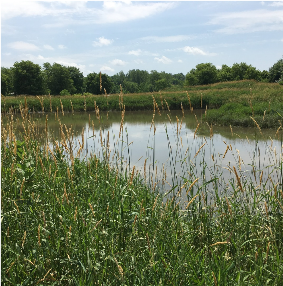
Figure 8. North silt pond, in need of renovation.
