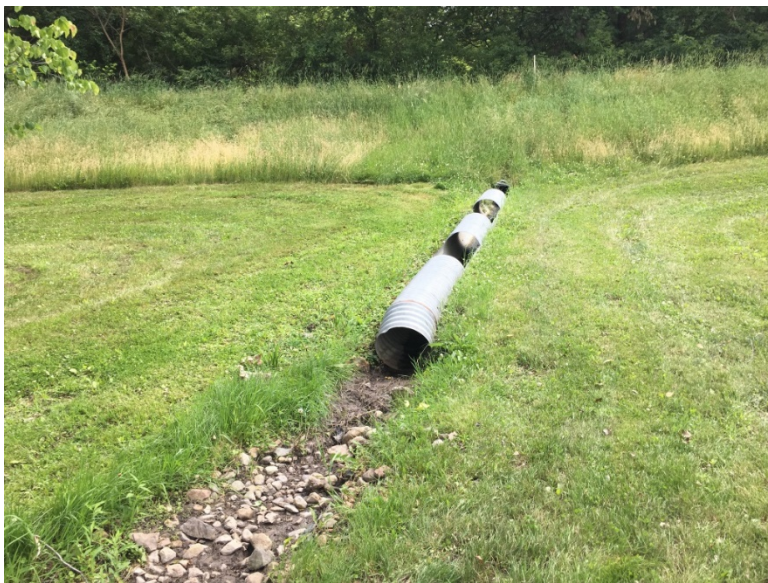
Figure 1 – Culvert draining to the north of the beach.
