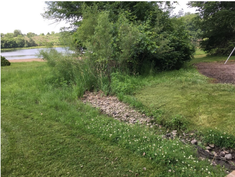
Figure 3. Outlet of the ditch along beach. This area could be repurposed to a wetland or LID feature to better treat water and improve drainage of this area.
