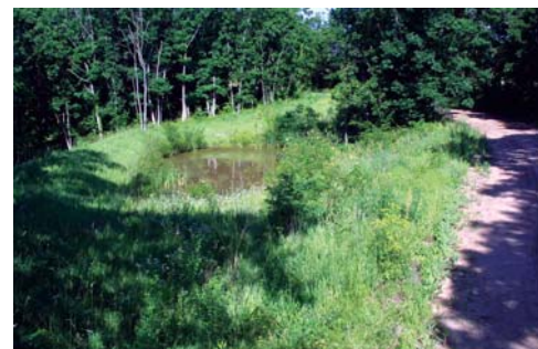
One of Nine Eagles State Park's many sediment retention basins.
