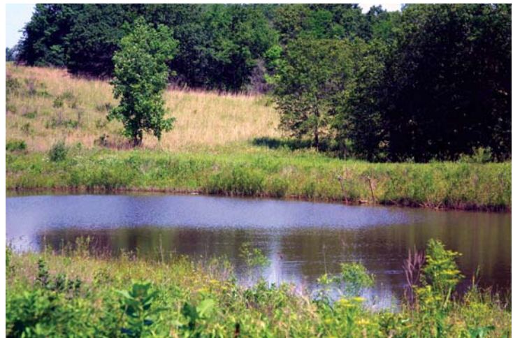
A sediment retention structure in Slip Bluff Lake Park.
