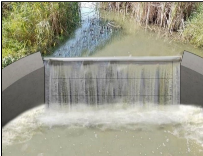
Figure 18 - Outlet Structure Modifications
