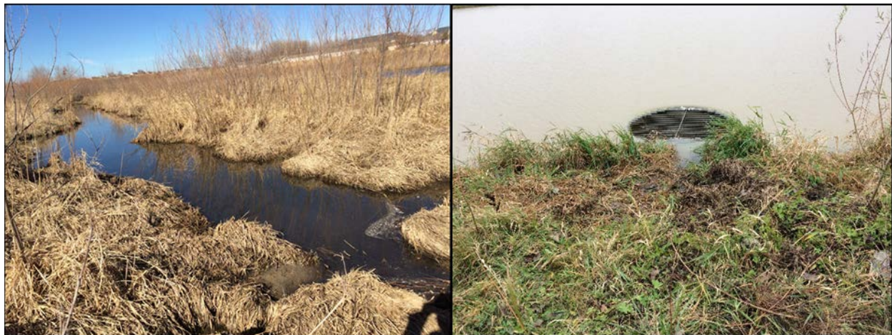
Figure 41. The image on the right is an example of a retention pond constructed in a new housing development in Cedar Falls. Retention ponds can be used to slow the rate of flow and artificially managing water, although the example on the right has a drain where the water would go down into the sewer system instead of flowing naturally into the stream or being infiltrated into the ground. The photograph on the left provides an example of a relatively successful restoration project; Located on UNI's campus, this wetland project is beginning to manage water effectively while providing positive influences on the Dry Run Creek and its overall health.
