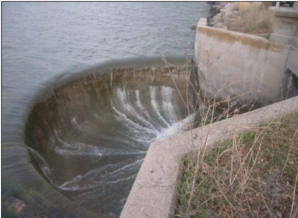
Figure 2-2. Discharge spillway at the east end of Black Hawk Lake.
