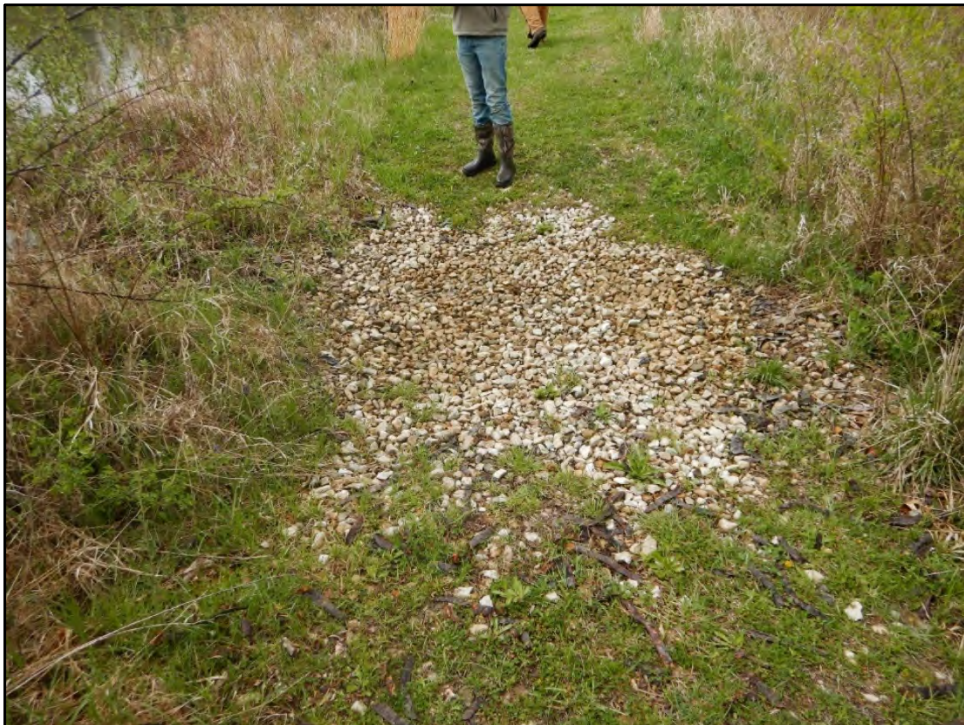
Figure 6: Photo taken on 4/20/21 showing earth cut auxiliary spillway.
