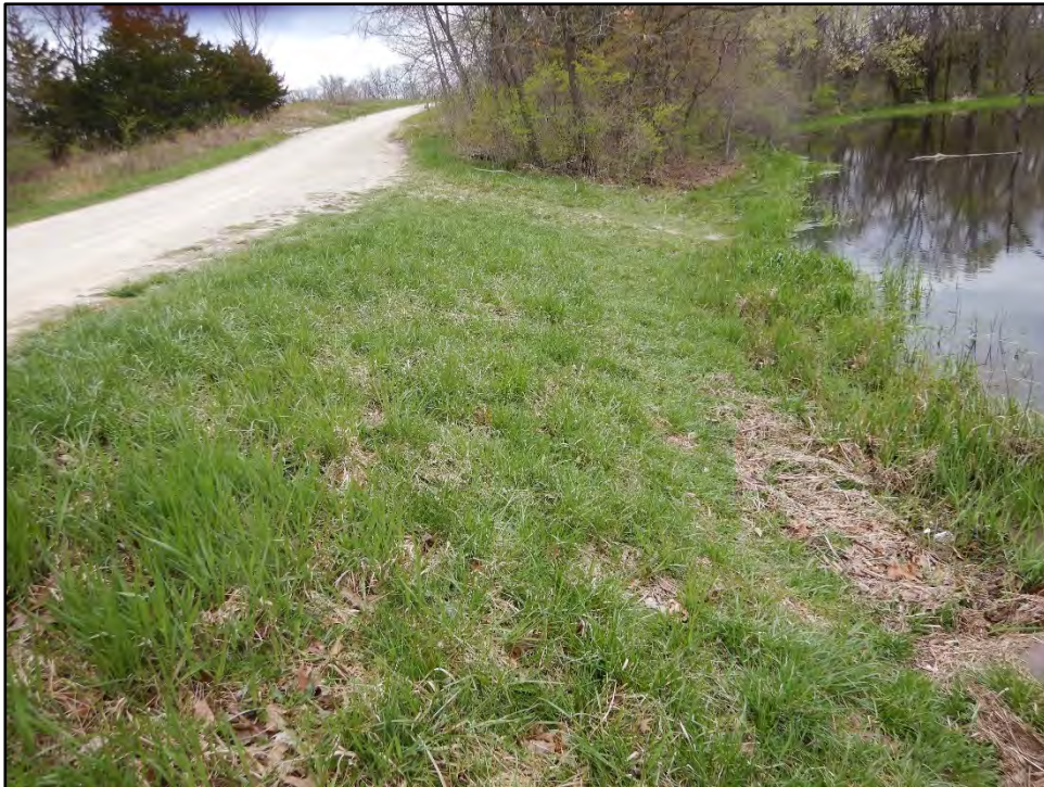
Figure 32: Photo taken on 4/20/21 showing the upstream slope of the dam.
