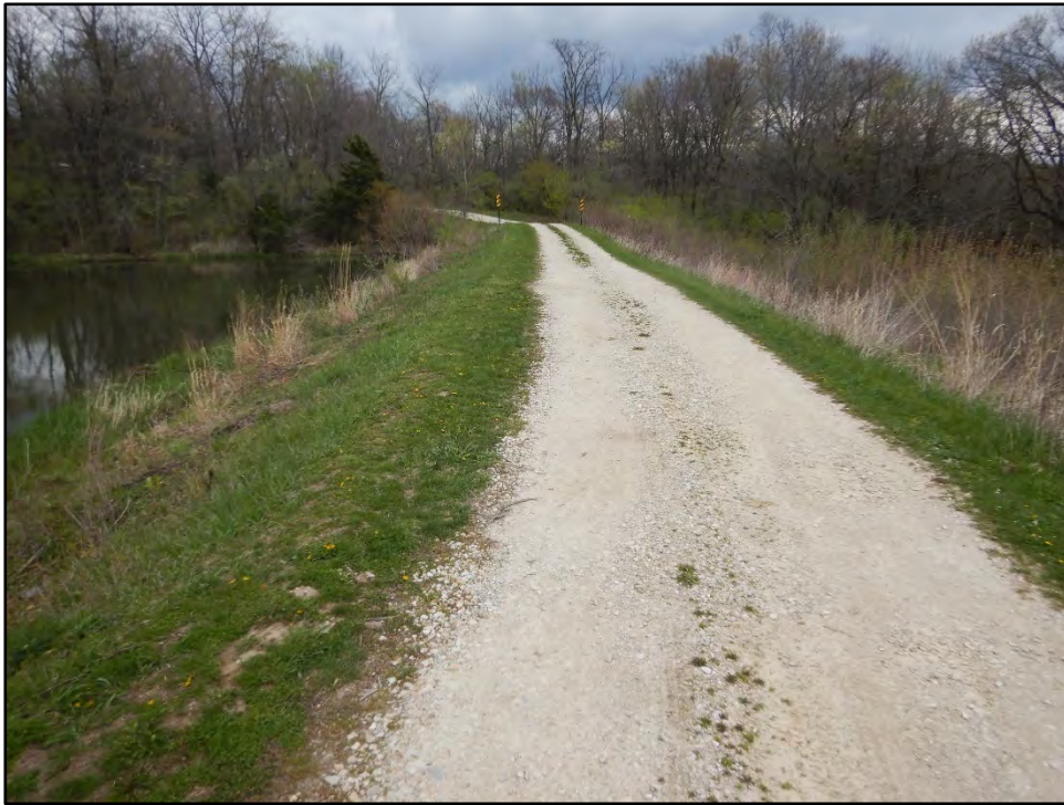
Figure 39: Photo taken on 4/20/21 showing the top of dam crest.
