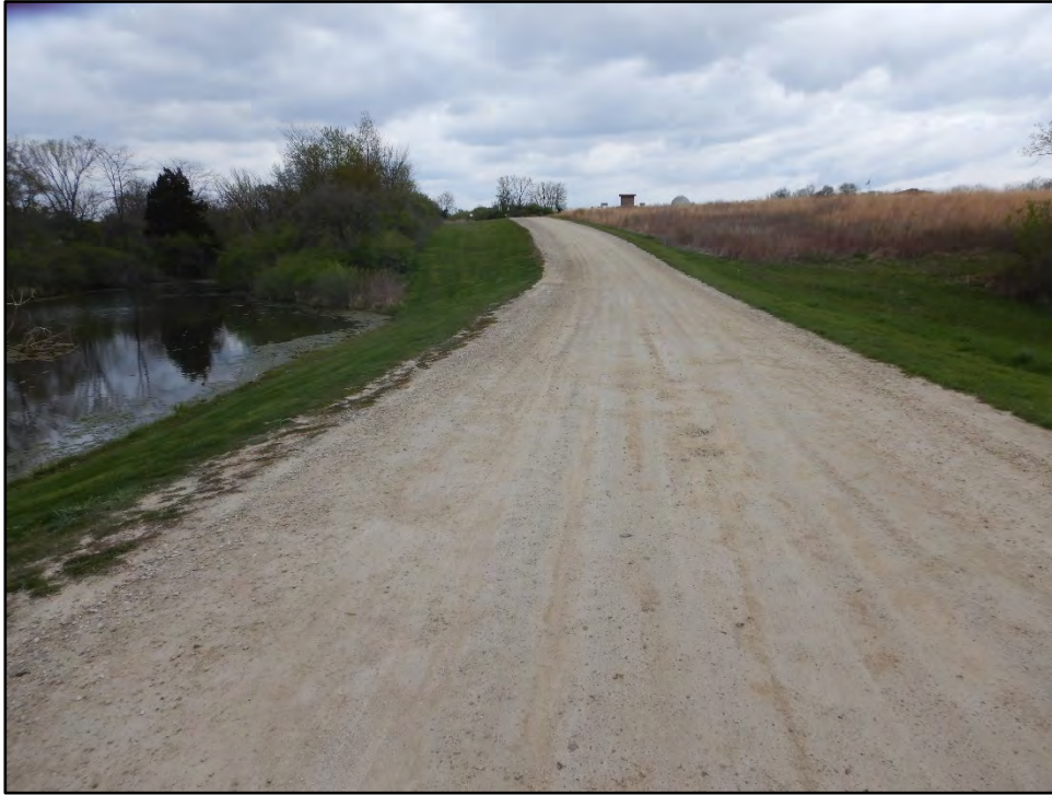
Figure 19: Photo taken on 4/20/21 showing the dam crest.
