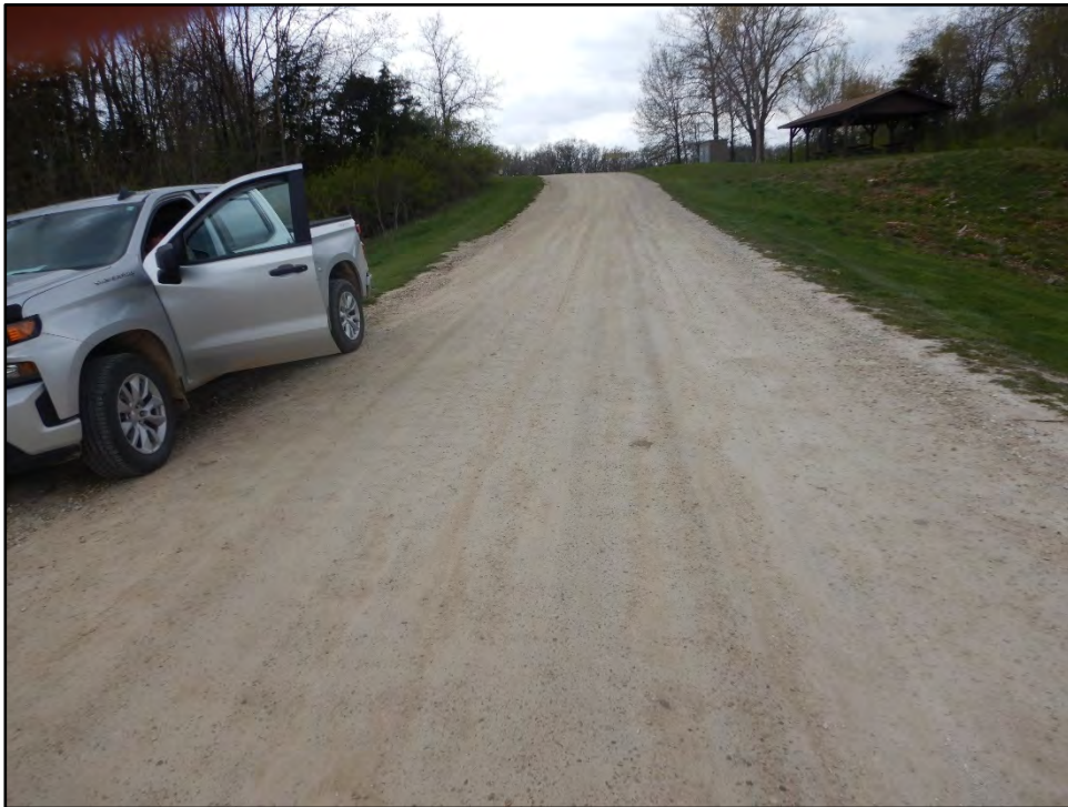
Figure 20: Photo taken on 4/20/21 showing the dam crest
