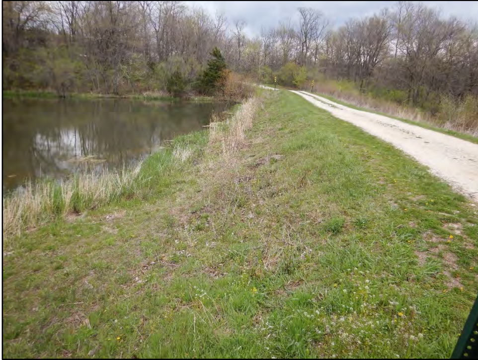
Figure 41: Photo taken on 4/20/21 showing the upstream slope of the dam.
