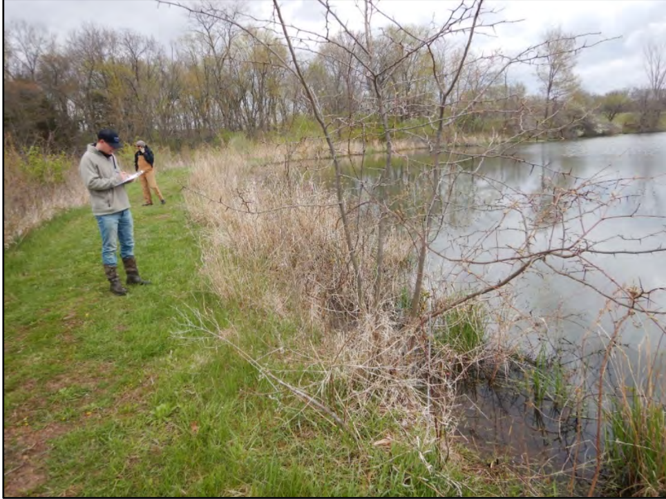
Figure 7: Photo taken on 4/20/21 showing trees growing at the water line.
