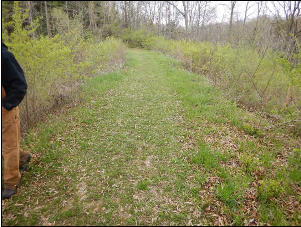
Figure 47: Photo taken on 4/20/21 showing the top of dam crest.
