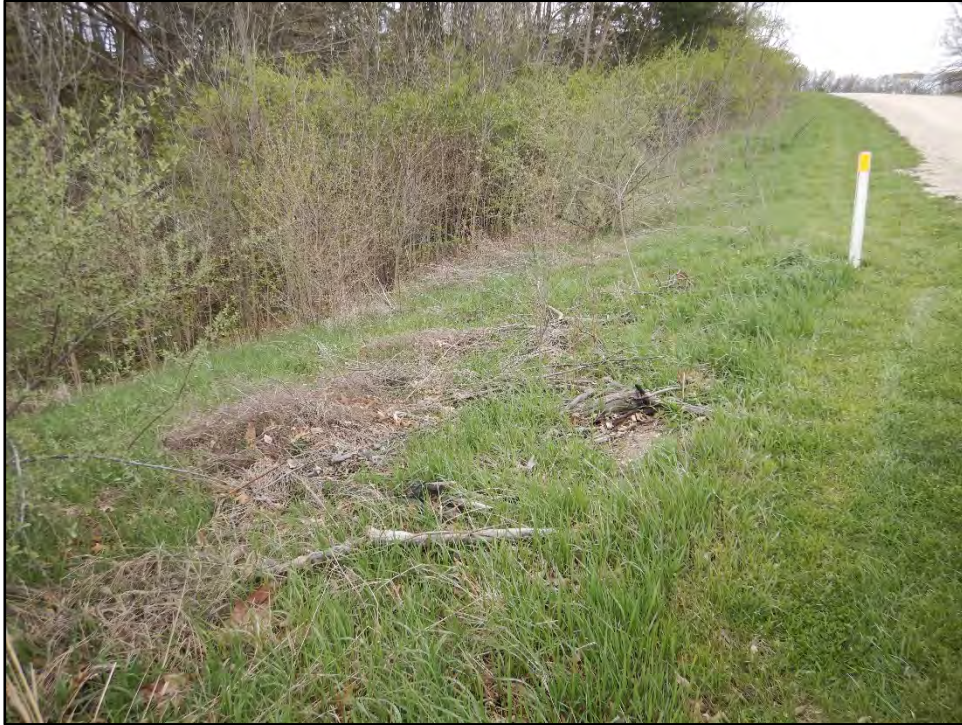
Figure 27: Photo taken on 4/20/21 showing minor trees and brush on the downstream slope of the dam.
