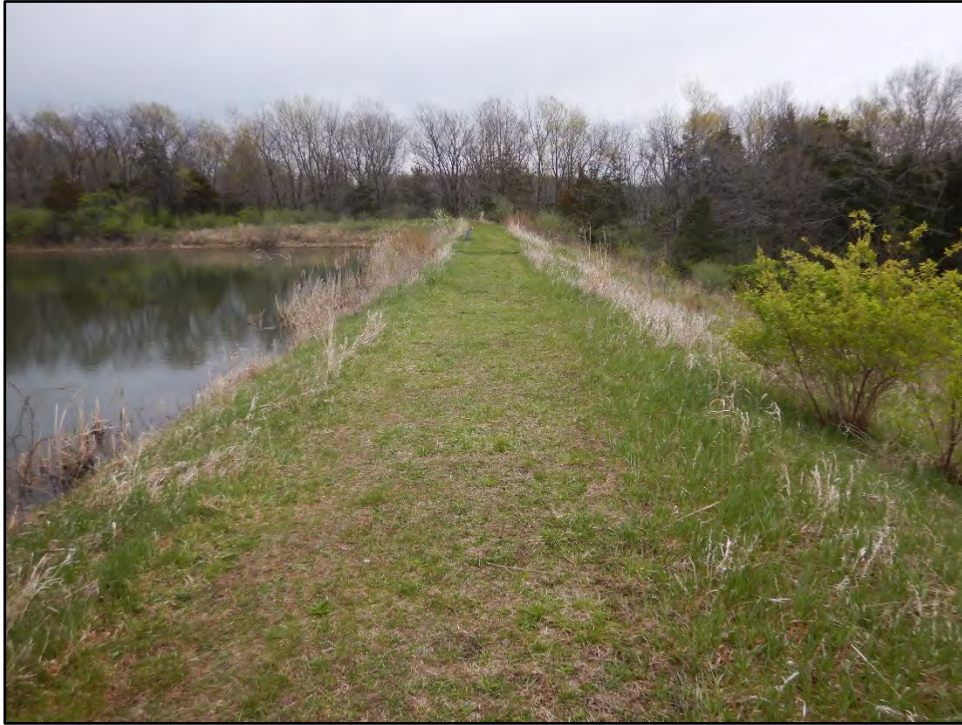
Figure 9: Photo taken on 4/20/21 showing the top of dam crest.
