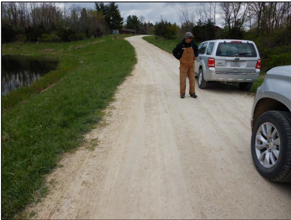
Figure 30: Photo taken on 4/20/21 showing the top of dam crest.
