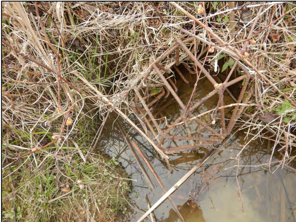
Figure 12: Photo taken on 4/20/21 showing 6" CMP principal spillway inlet with rebar trash rack.
