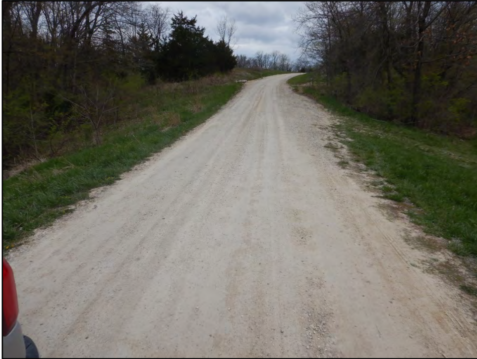
Figure 29: Photo taken on 4/20/21 showing the top of dam crest.
