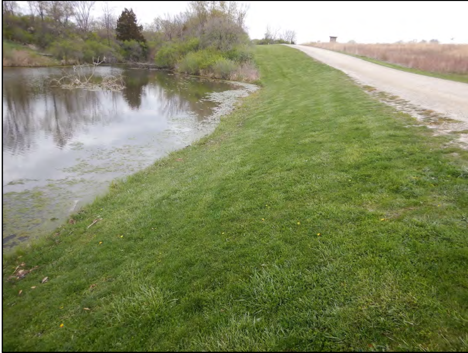
Figure 21: Photo taken on 4/20/21 showing the upstream slope of the dam.
