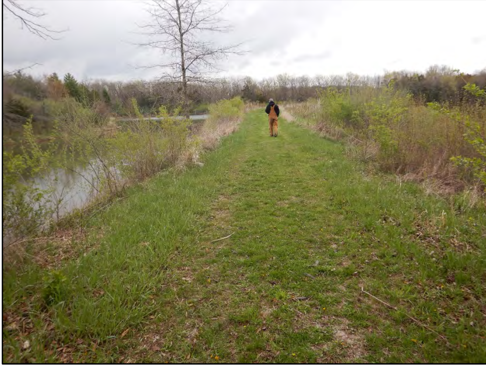
Figure 17: Photo taken on 4/20/21 showing trees and brush growing at water line
