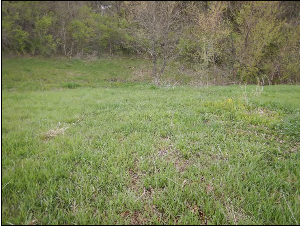
Figure 23: Photo taken on 4/20/21 showing the downstream slope of the dam.
