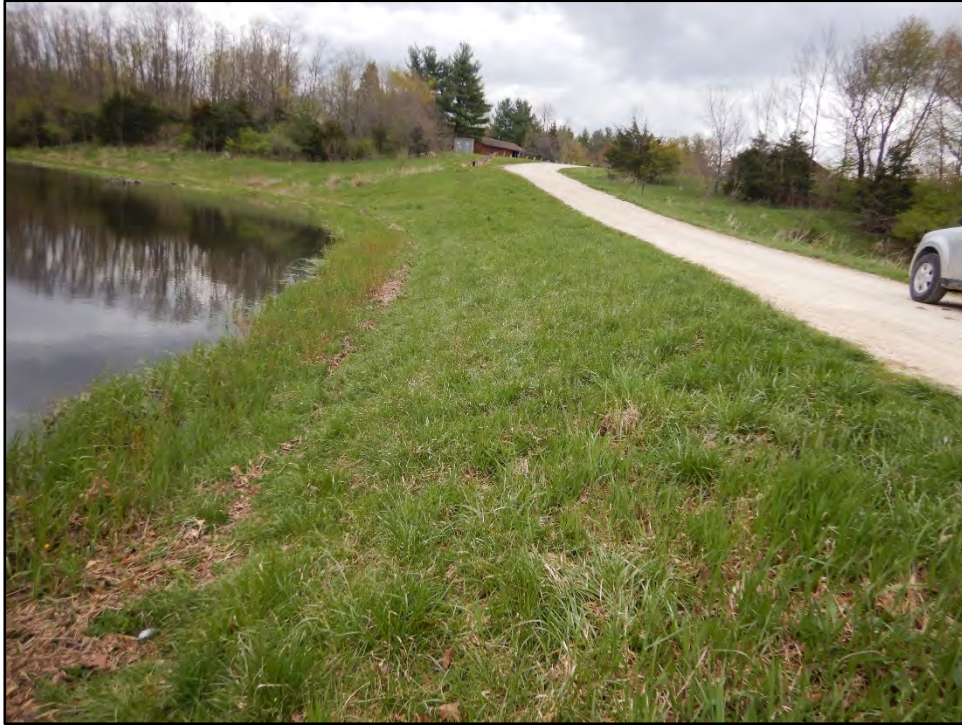
Figure 31: Photo taken on 4/20/21 showing the upstream slope of the dam.
