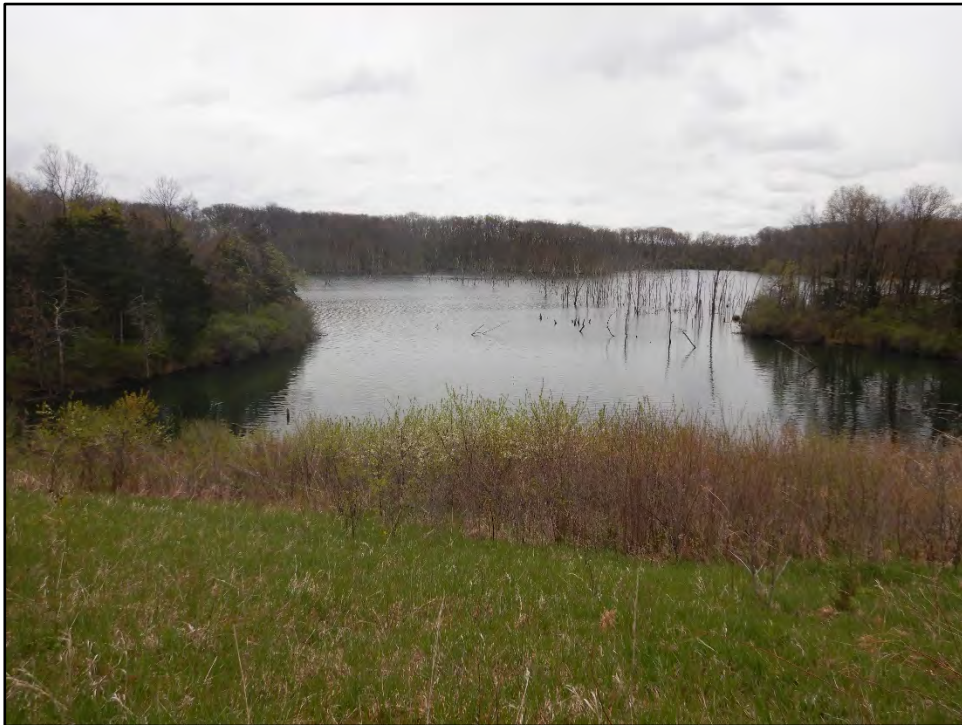
Figure 10: Photo taken on 4/20/21 showing trees and brush growing on downstream slope.
