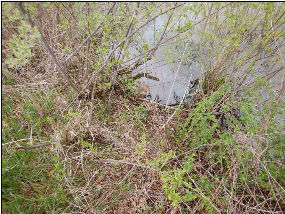
Figure 50: Photo taken on 4/20/21 showing the 6" CMP with hooded inlet.
