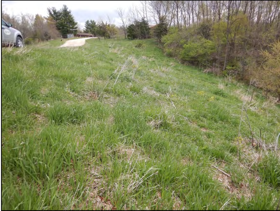
Figure 33: Photo taken on 4/20/21 showing the downstream slope of the dam.
