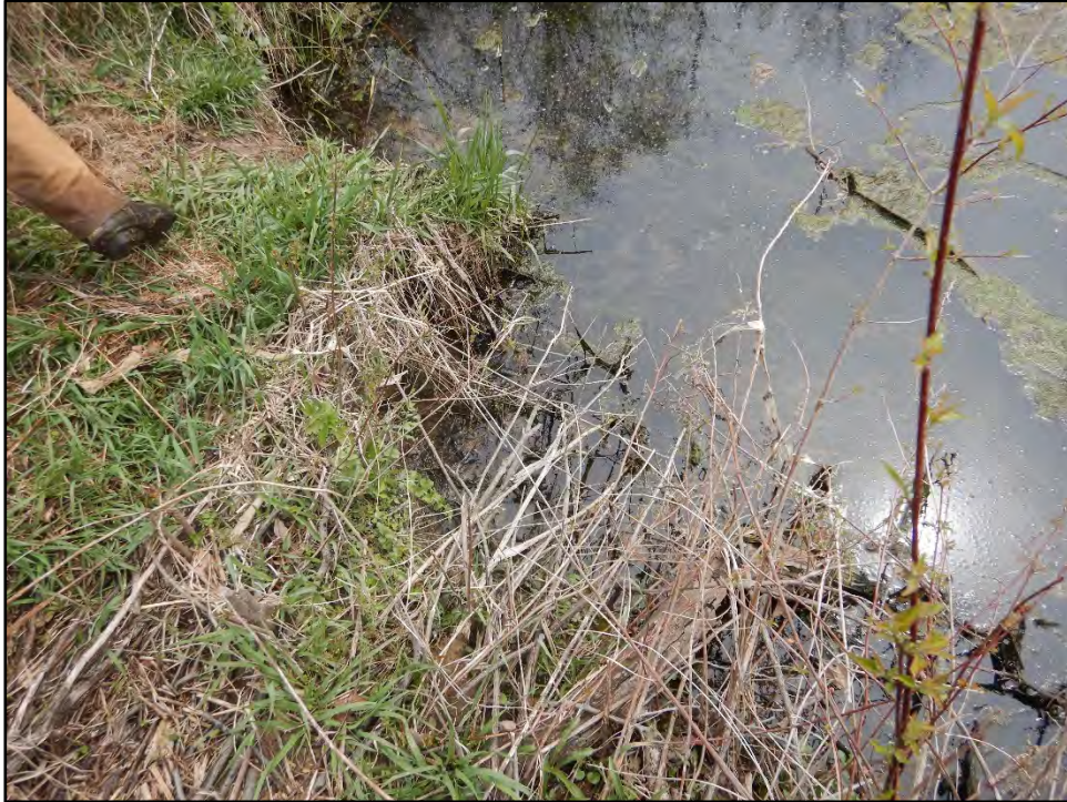
Figure 13: Photo taken on 4/20/21 showing approximate location of submerged principal spillway outlet.
