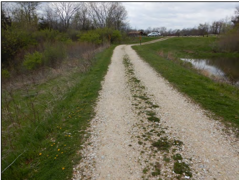
Figure 40: Photo taken on 4/20/21 showing the top of dam crest.
