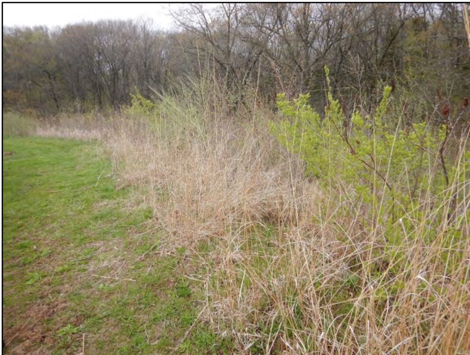
Figure 2: Photo taken on 4/20/21 showing the trees and brush growing on downstream slope of the dam.
