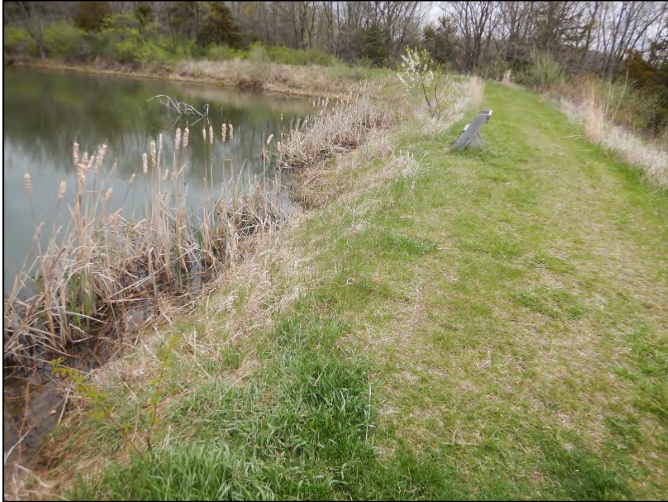
Figure 11: Photo taken on 4/20/21 showing the upstream slope of the dam.
